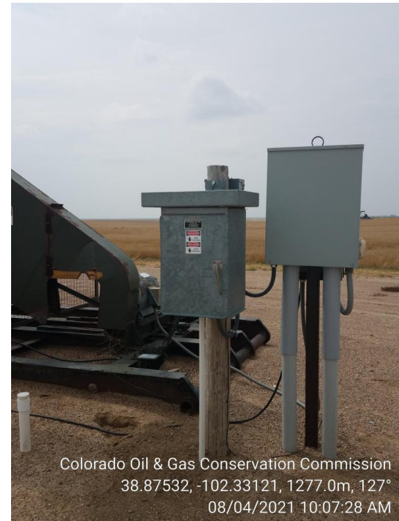
2. Elec panels, Cathodic rectifier, Prime Mover
