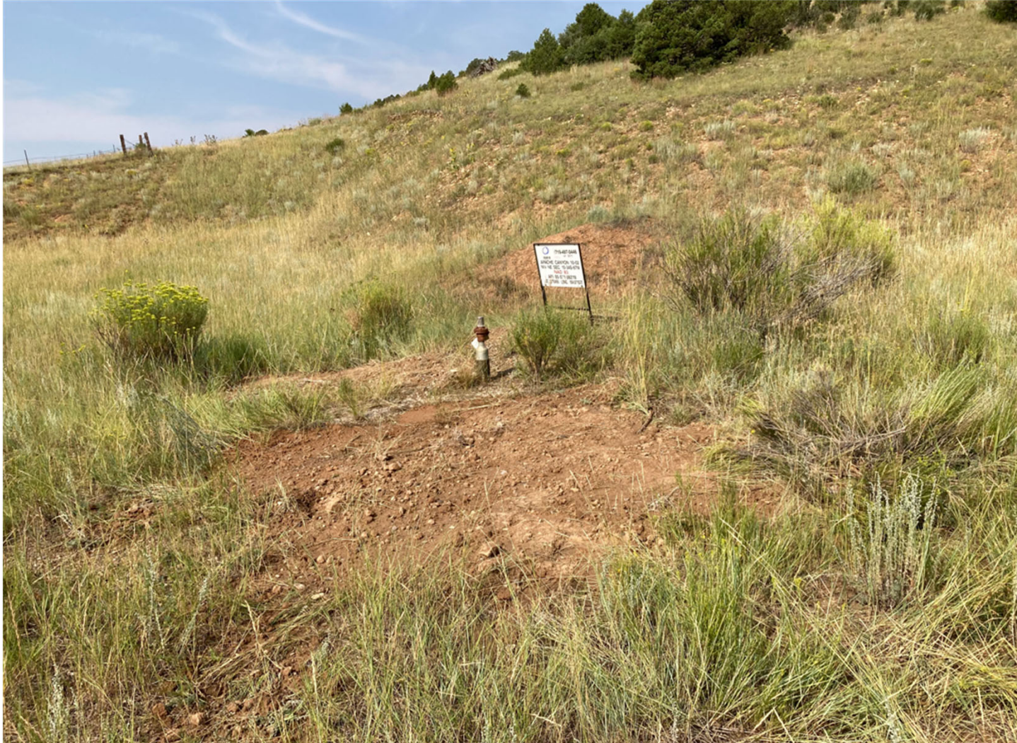
PHOTO 1: THE WELL HEAD RISER WAS LOTO. THE REMAINING RISERS WERE REMOVED FROM THE LOCATION.
