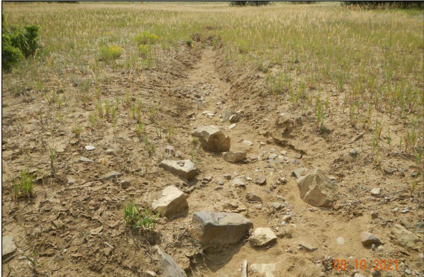
Photo 3. View of southwestern diversion channel, where erosional down-cutting is occurring. Stabilization measures are needed here.
