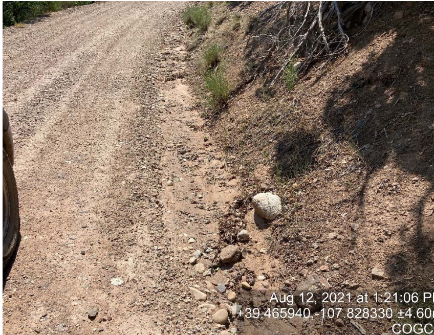
Ditch on access road failing
