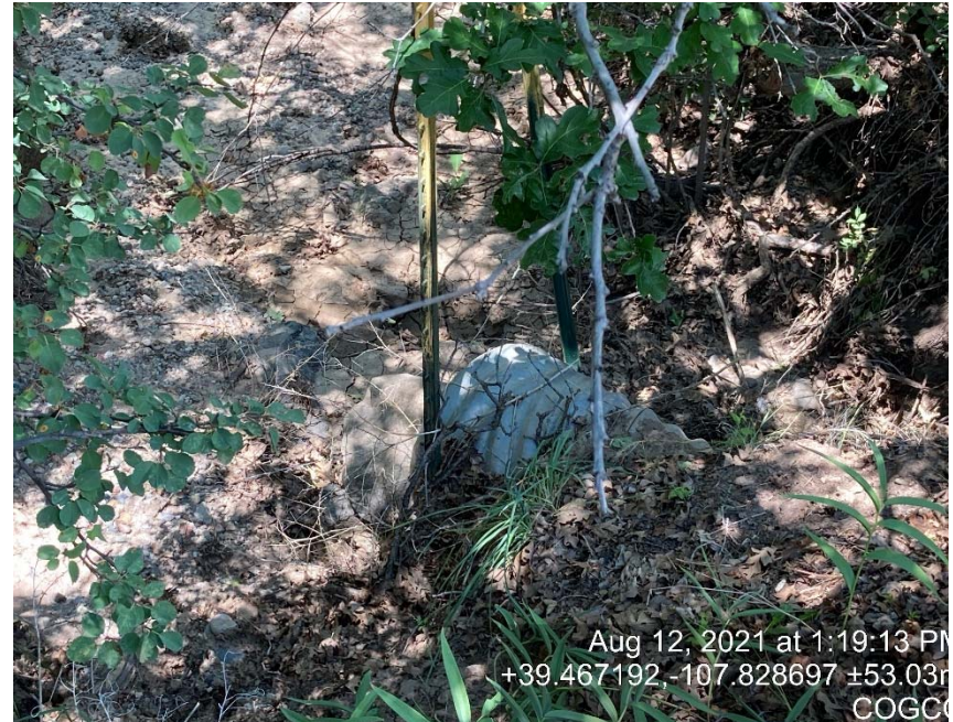
Culvert outlet from completely buried inlet side
