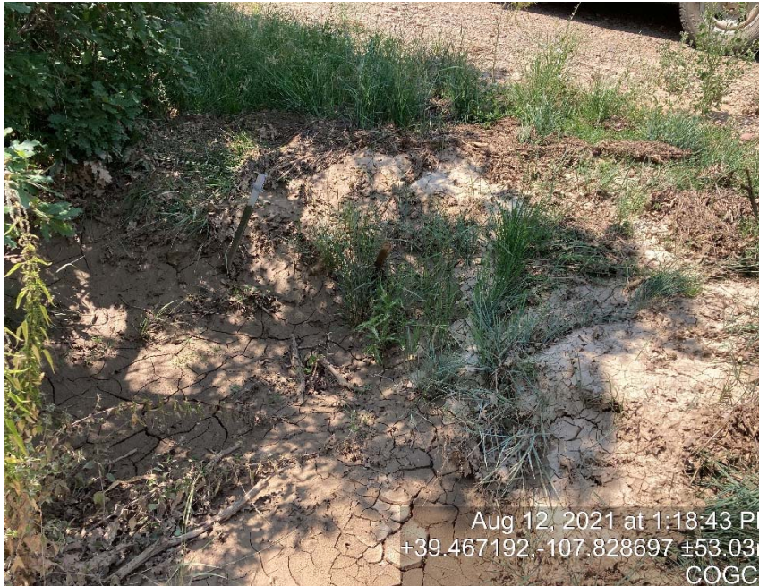
Culvert inlet failing/completely buried
