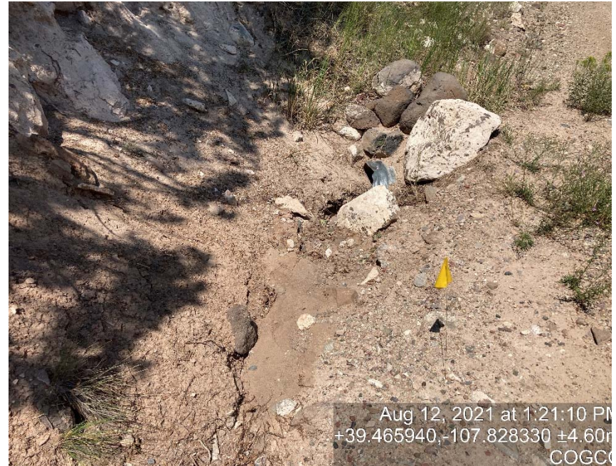
Culvert inlet failing
