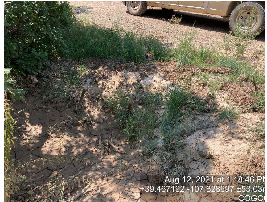
Culvert inlet failing/completely buried
