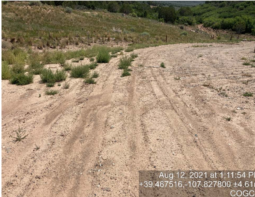
Lack of stabilization/compaction/weeds
