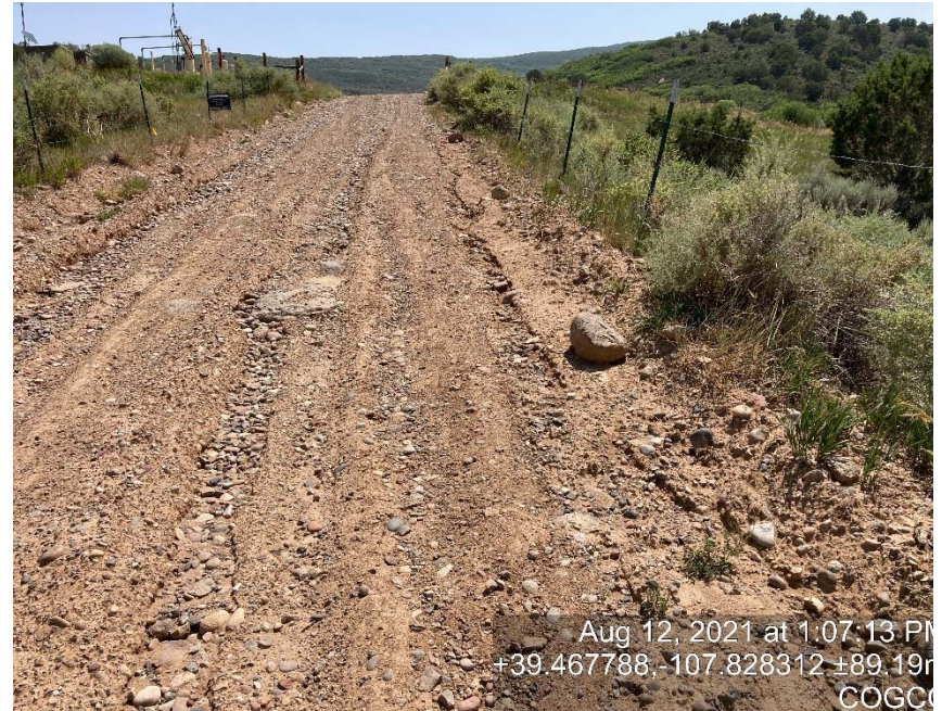
Access road lack of stabilization/compaction/erosion
