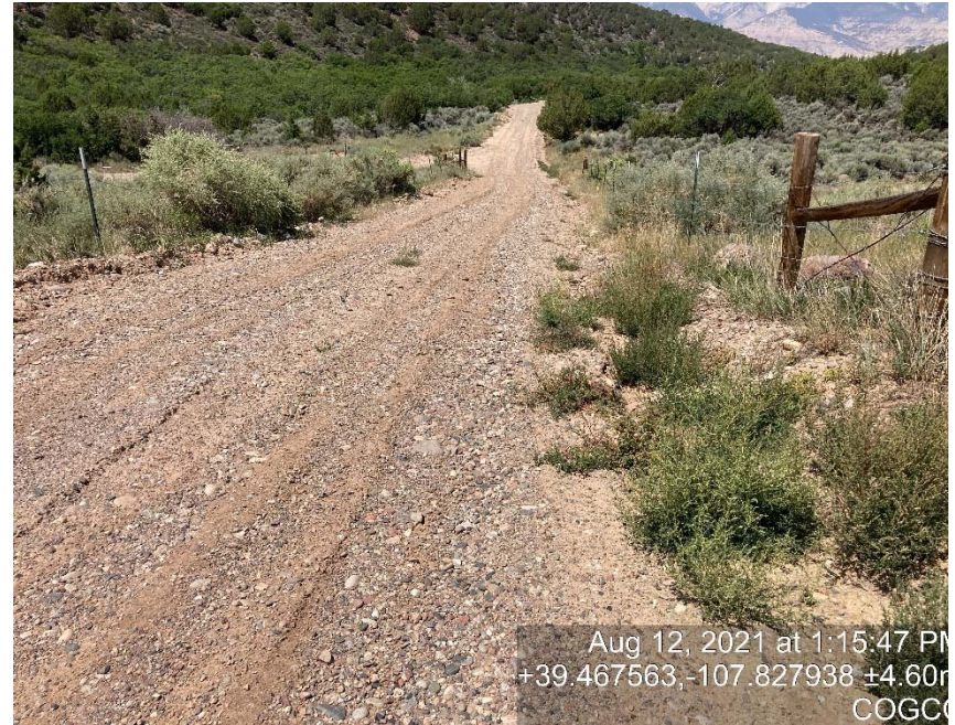
Access road lack of stabilization/compaction/erosion
