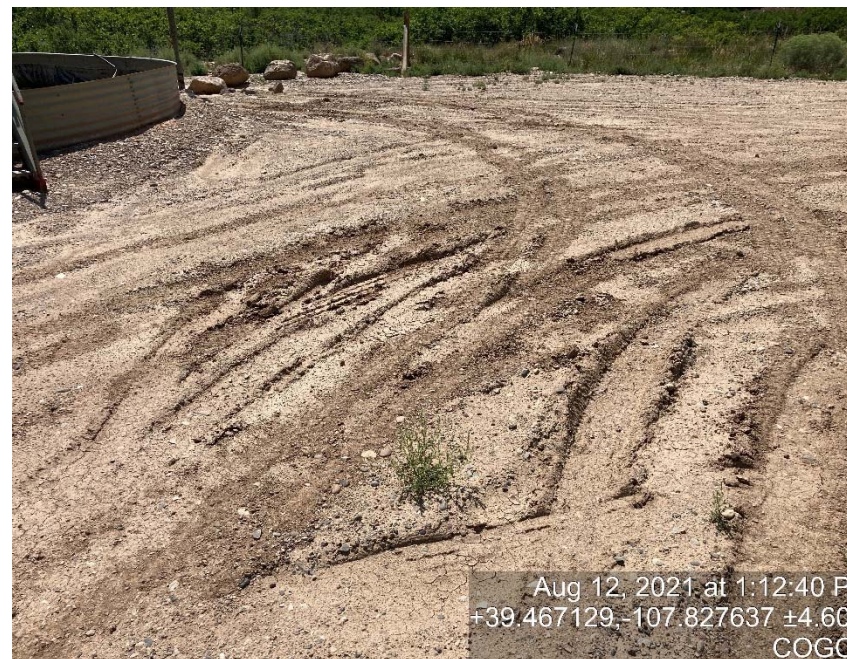
Lack of stabilization/compaction
