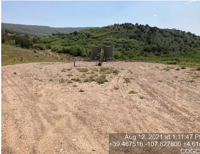
Lack of stabilization/compaction/weeds
