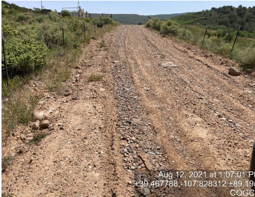
Access road lack of stabilization/compaction/erosion
