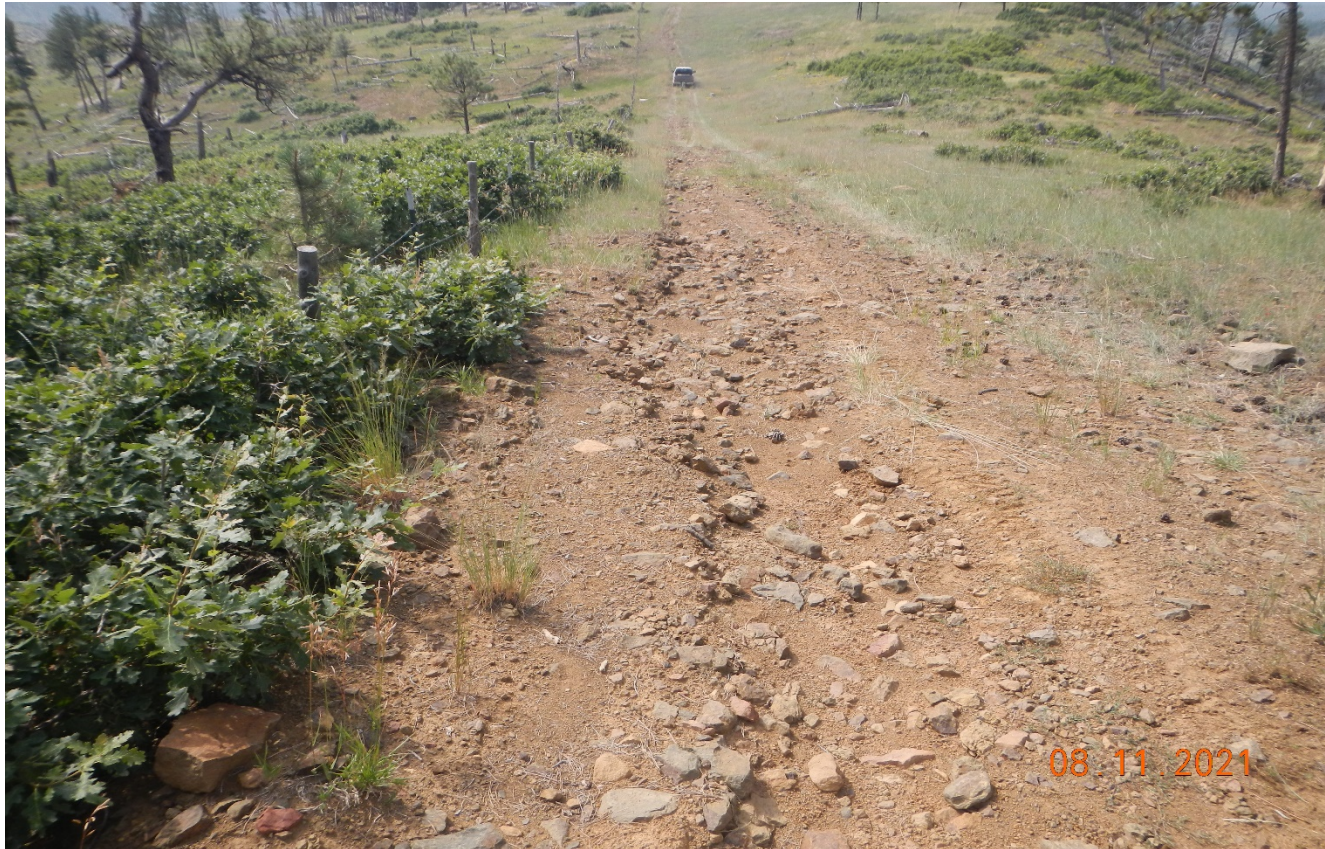
Photo 1. Facing south along the pre-existing access road. There is erosion occurring down the road. Stormwater is not being diverted off the road which will continue to cause erosion. BMP's are needed to control stormwater erosion in this area..
