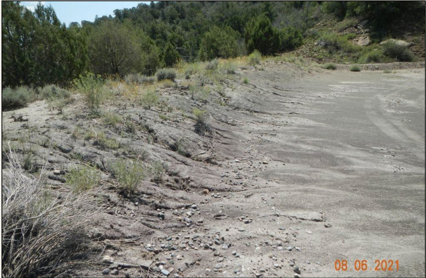
Photo 2. View of the eastern cutslope facing southward. Erosional channeling and rilling up to 1-foot deep observed, with sediment deposition at the toe of the unstabilized slope.
