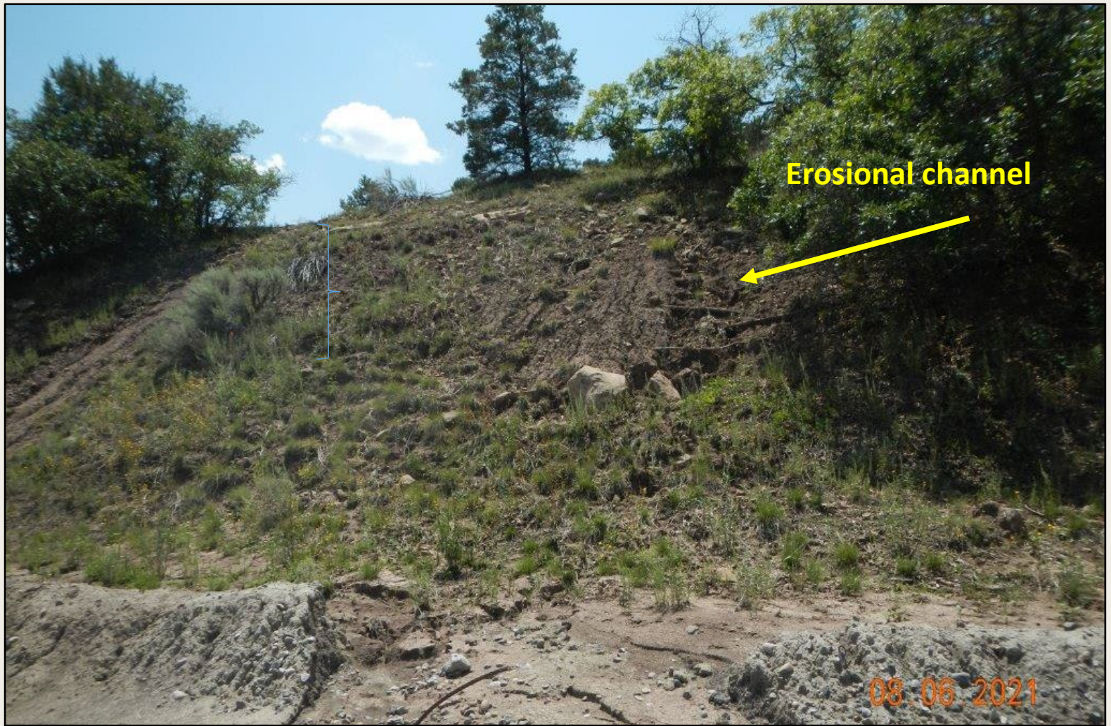
Photo 3. View of erosional channel within the southern project area, and area where diversion berm is breached. Rilling observed across slope and diversion channels are full of sediment.
