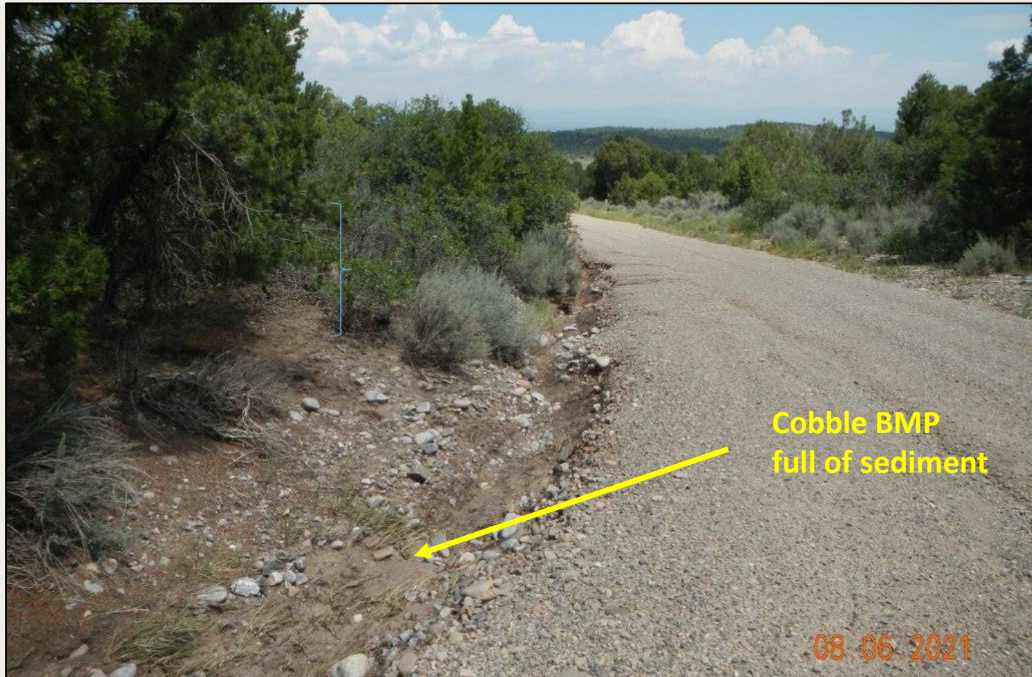
Photo 5. View of area along the access road where cobble BMPs are full of sediment and scouring is occurring. These BMPs are not adequate here.
