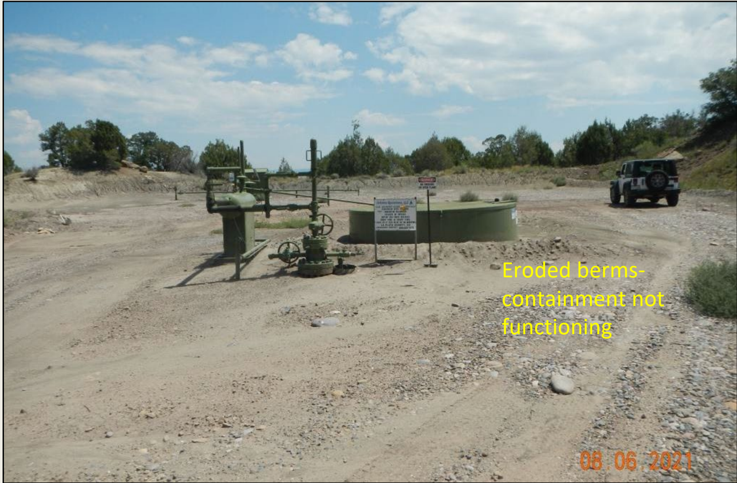
Photo 1. View of the project area from the well pad entrance facing center. Containment berms around submerged tank are eroded and no longer functioning.
