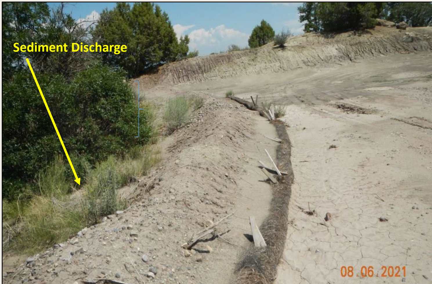
Photo 4. View of berms and wattles within the northern project area. Berms are not stabilized and sediment is discharging down slope (offsite).
