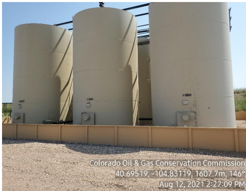
Photo 3: Tank Battery
