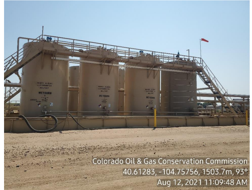
Photo 2: Tank Battery
