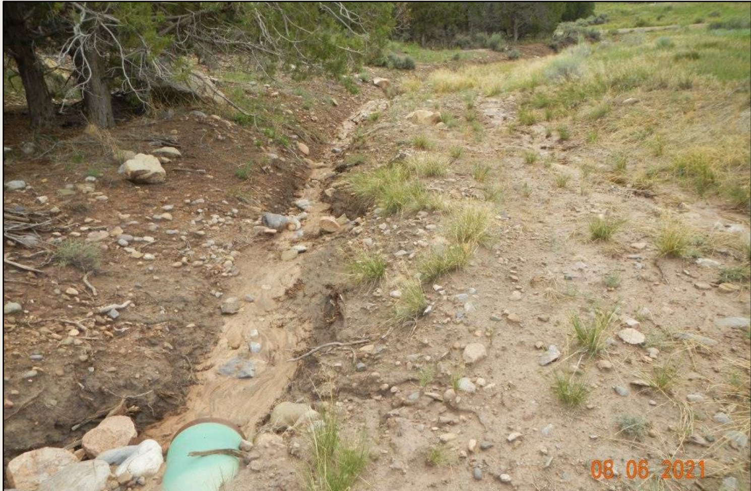
Photo 6. View of stormwater diversion within the northeastern well pad. Stormwater controls are needed to reduce velocity and stabilize soils when stormwater flows exit the culvert and flows down-slope away from the project area.
