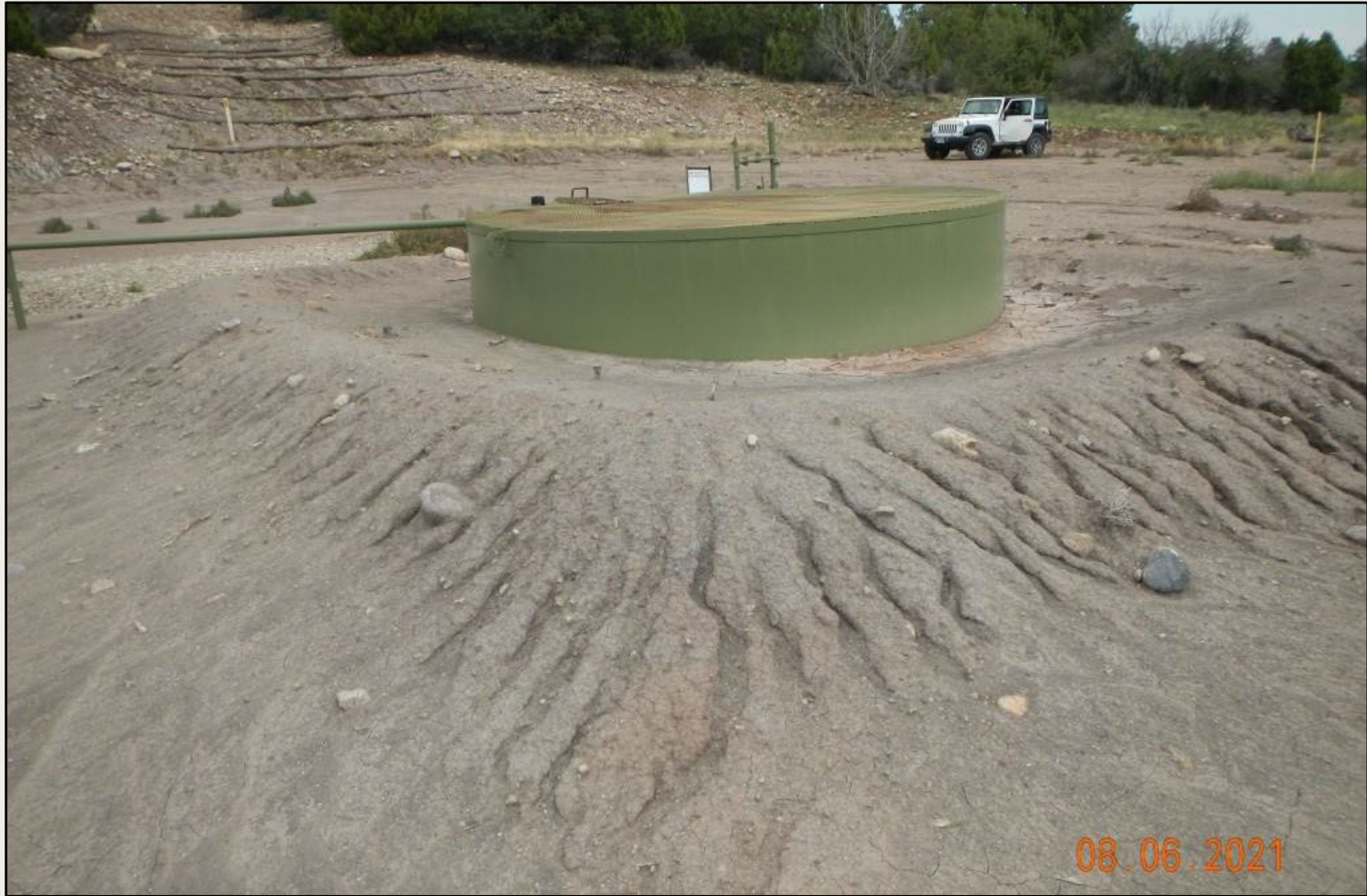
Photo 5. View of eroding berms and in tank containment. Sediment accumulation within containment is resulting in reduced and inadequate containment volume. Berms are not stabilized.
