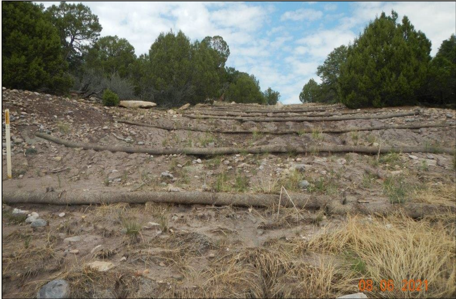
Photo 3. View of erosional channeling and rilling where flowline right of way overlaps the northwestern cut-slope. Wattles are not functioning and are not an adequate BMP in this area.
