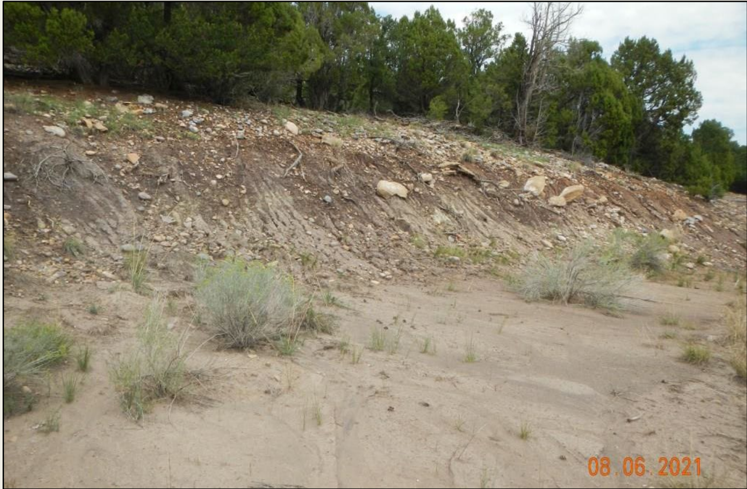
Photo 2. View of erosional rilling and sediment deposition within the western cut-slope. Area needs erosion controls, run-on, and sediment controls installed and maintained until stabilized with long term perennial vegetation.
