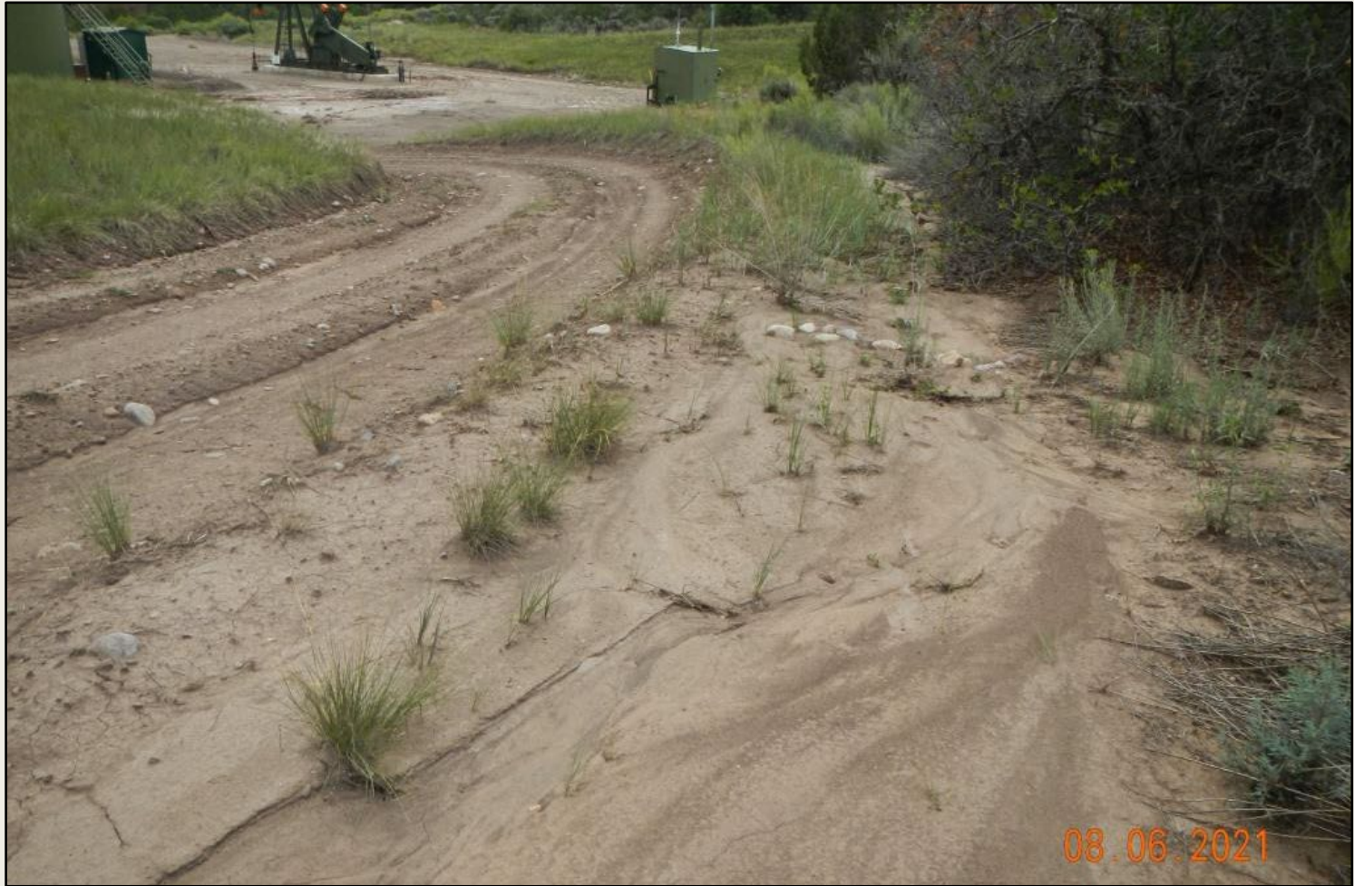
Photo 4. View of sediment discharge along the access road and cobble BMPs inundated with sediment. These cobble BMPs are not adequate for this area.
