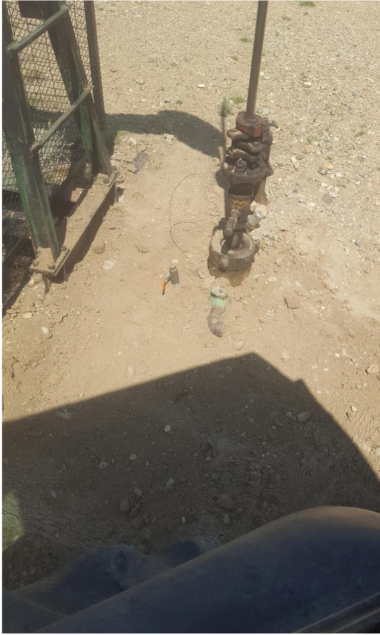
Figure #1 Bradenhead access has been installed.
