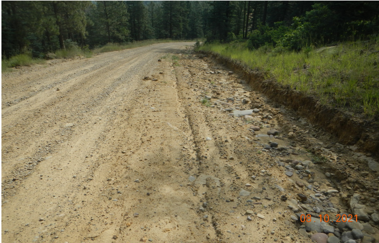
Photo 4. Facing back down the road. The erosion along the road was graded but no BMP's were installed on the long stretch of road to prevent erosion from reoccurring.
