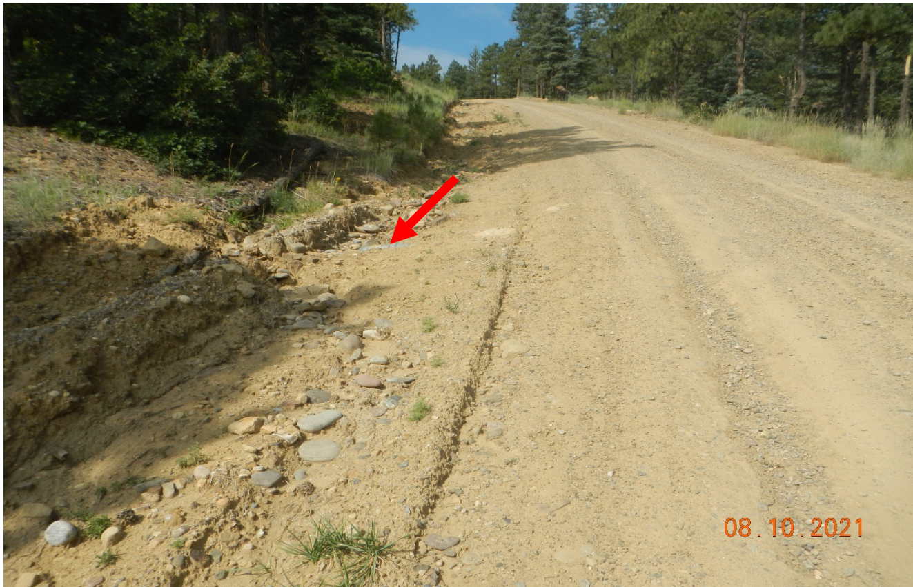
Photo 3. The erosion along the side of the road was repaired but no BMP's were installed to prevent erosion. Arrow points to a buried culvert that would help control erosion if repaired.
