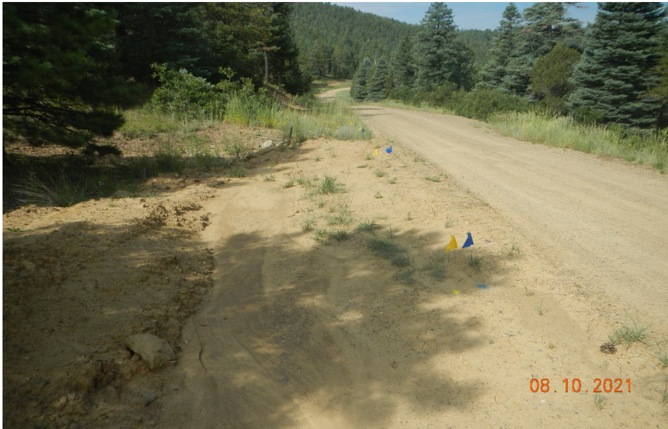
Photo 2. The culvert has been cleaned out and grading was performed to direct stormwater toward the culvert.
