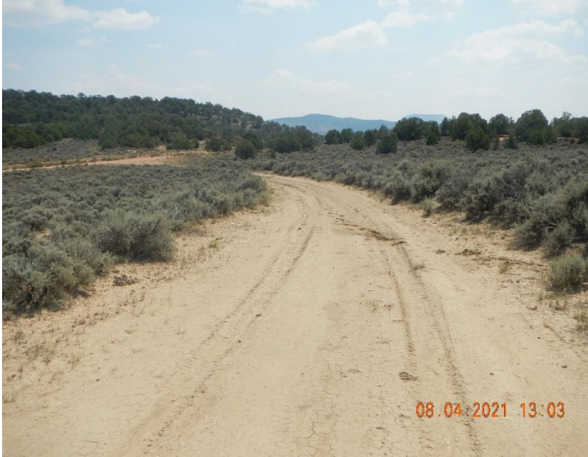
Rutting and movement of sediment on access road.
