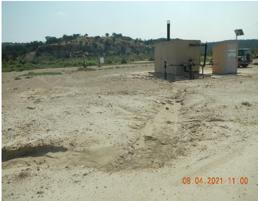
Storm water washing off location at meter shed and separator.
