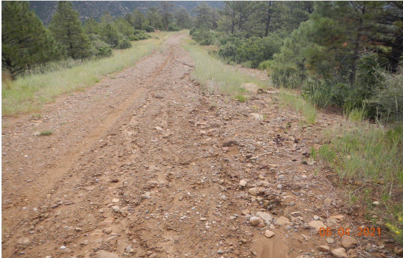
Photo 2. Facing back to the southeast t approx. Lat/Long:37.2217,105.00145. Stormwater is directed down the slope of the road causing erosion.
