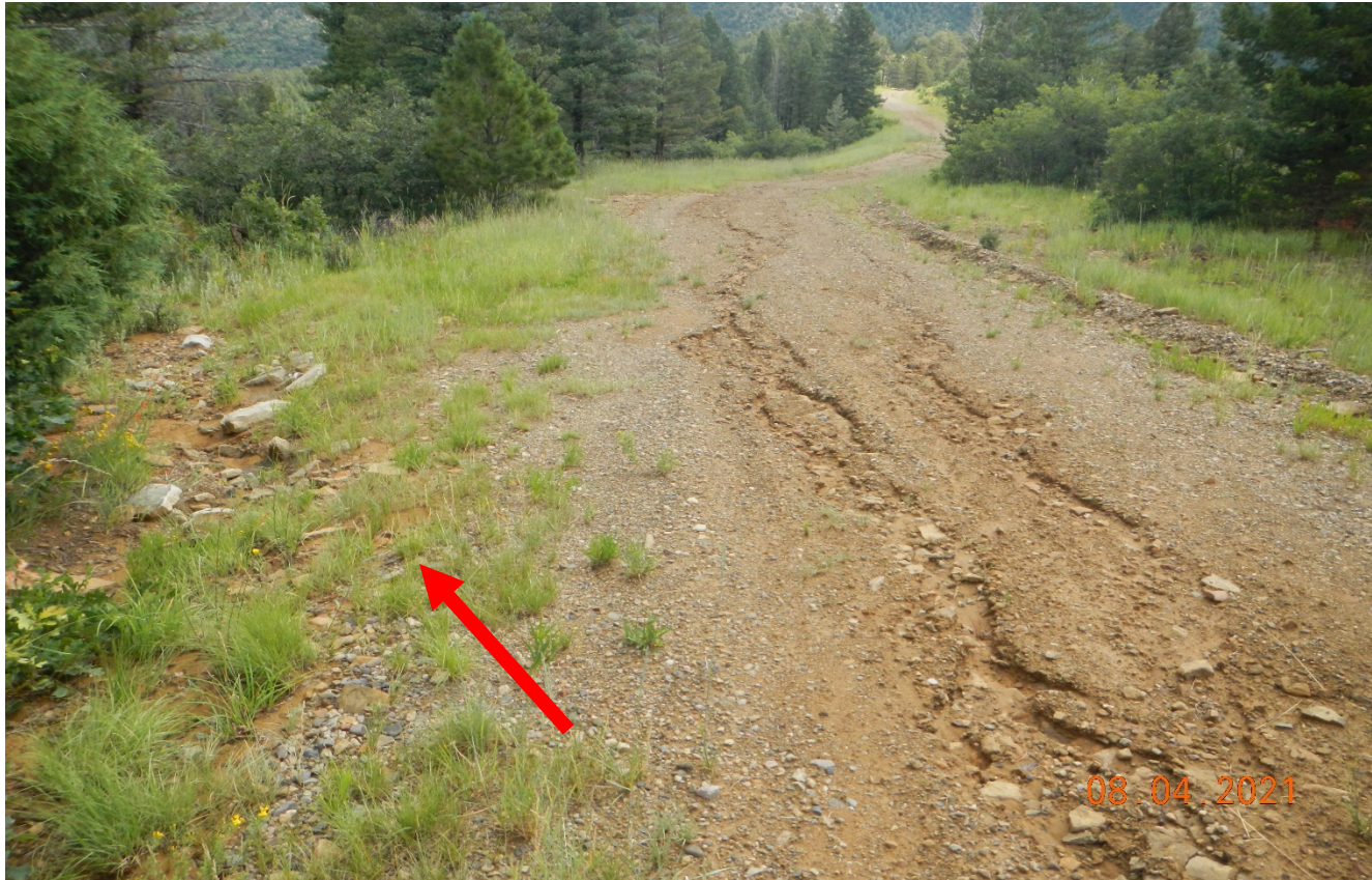
Photo 3. Same issue was observed at Lat/Long:37.22389,-105.00066. Stormwater should be directed off the road.
