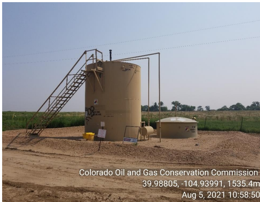
Photo 5 TNK BTRY Battery sign missing
