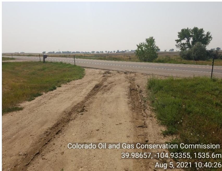
Photo 1 No tracking pad onto HWY 7 from well site.
