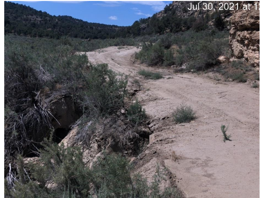
Erosion of access road. Washing away roadway.
