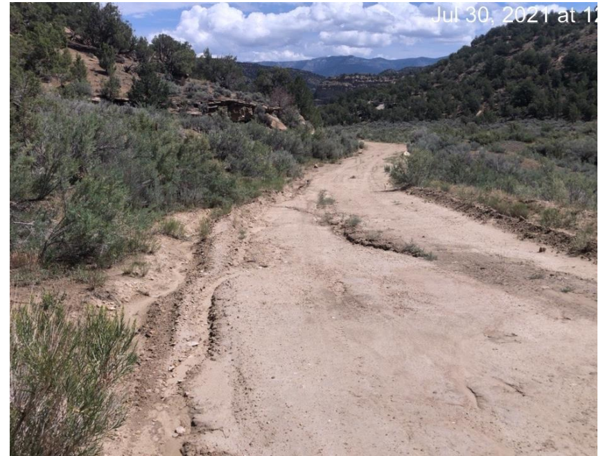
Erosion of access road.
