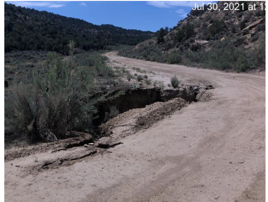
Erosion of access road. Washing away roadway.
