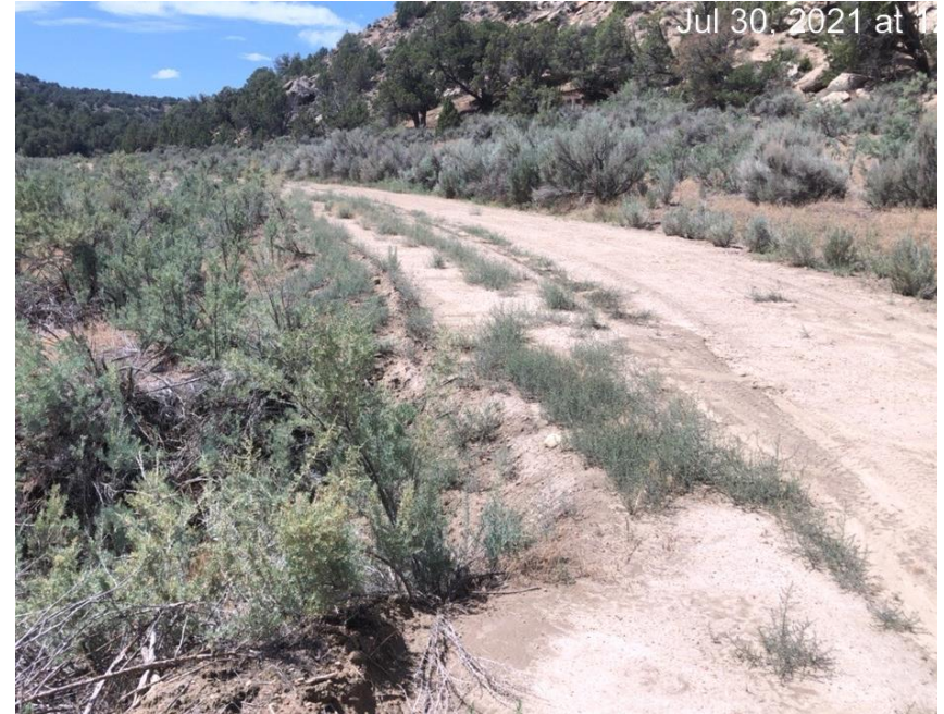
Erosion of access road. Washing away roadway.
