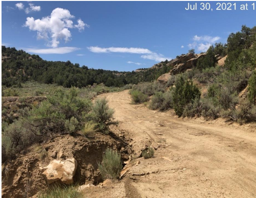
Erosion of access road. Washing away roadway.
