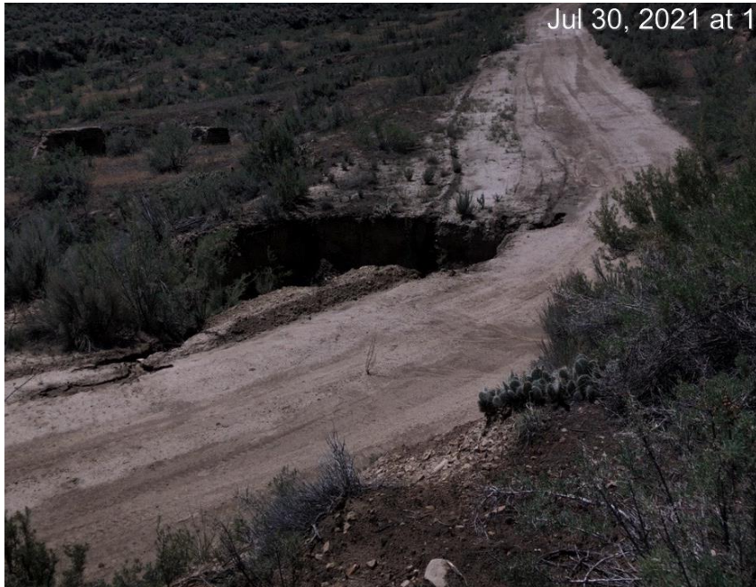
Erosion of access road. Washing away roadway.
