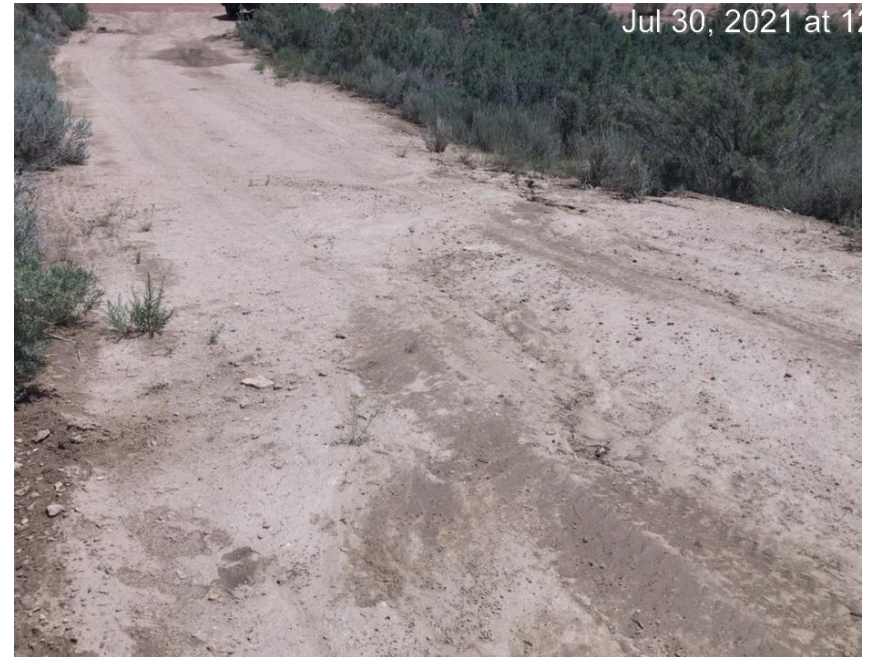
Movement of sediment across access road.
