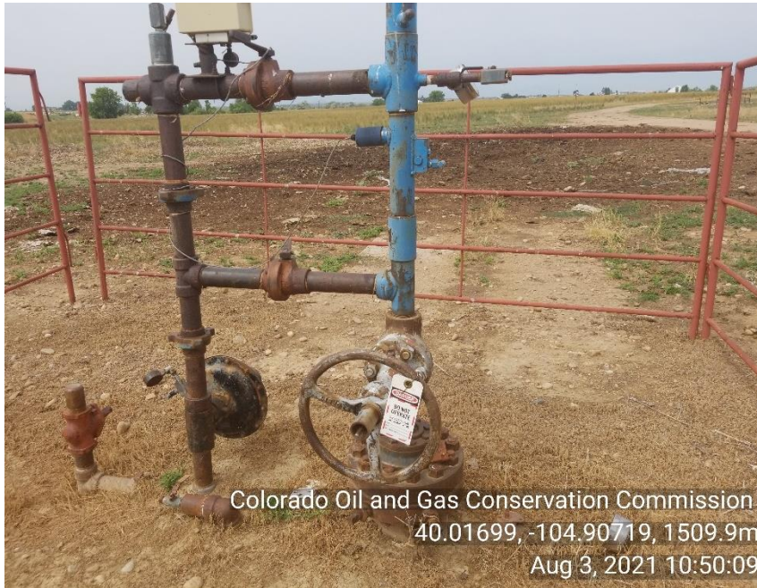
Photo 6 Well head id tagged out.
