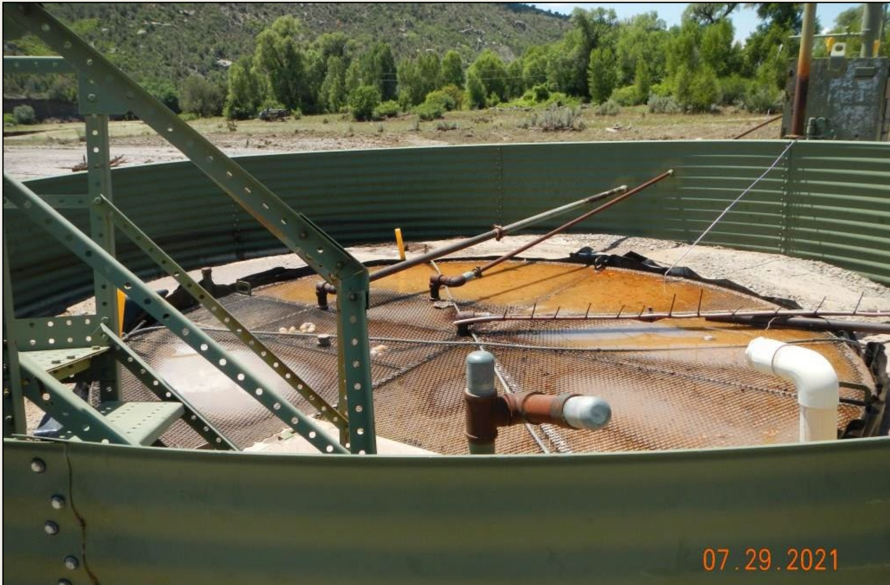
Photo 5. View of open tank full of liquid and bubbling, appears to be overflowing. Debris is floating in tank material and sediment deposition observed.
