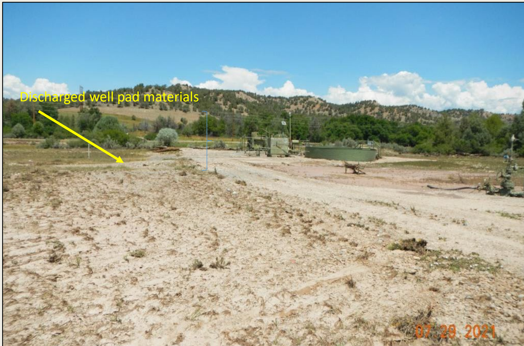
Photo 1. View of the location from the southwestern corner facing center. Flood event has washed well pad material off of well pad and deposited down-slope and likely downstream. Water flow is from right to left here.
