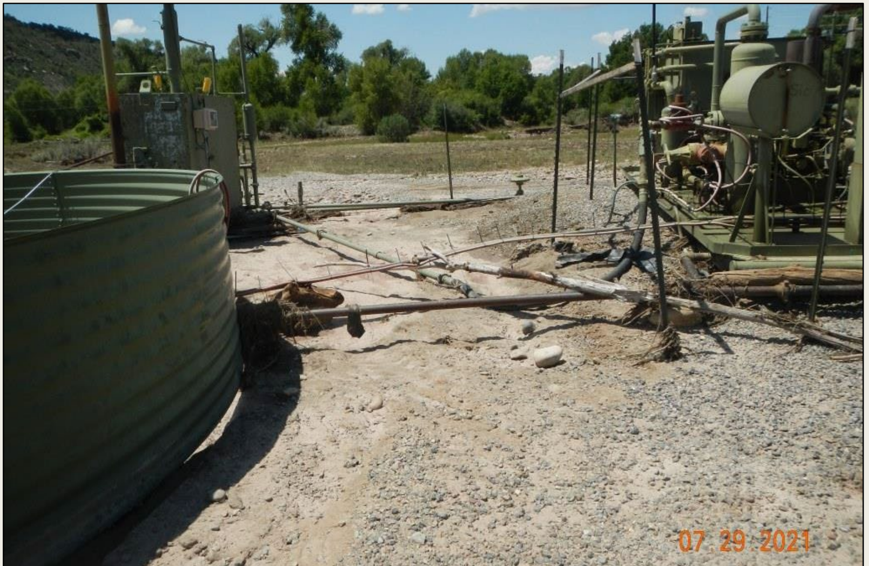
Photo 9. View of area with significant substrate loss exposing pipe and equipment infrastructure with large woody debris.
