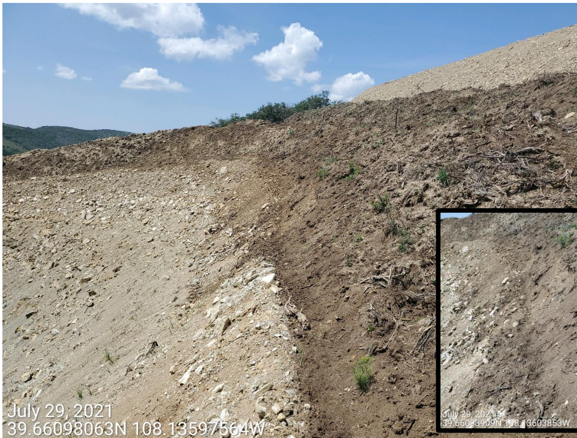
Photo 3: Photo taken on the North end of the Location. Photo shows example of slopes on the Location (cut/fill, and topsoil), where BMPs remain missing or insufficient to protect/stabilize. Darker soils on right is topsoil stored above a cut slope; hydromulch on topsoil no longer in proper functioning condition.
