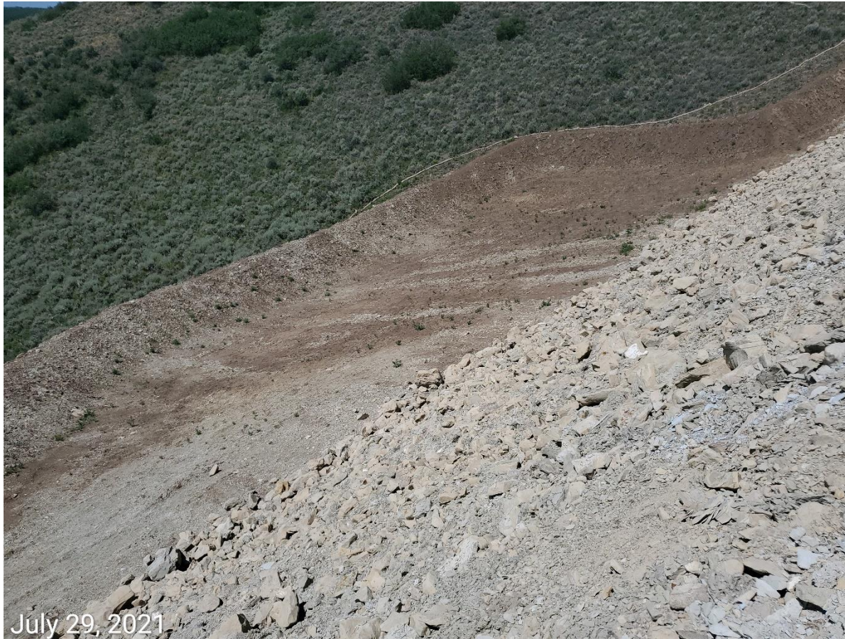
Photo 5: Photo taken from the the west end of the Location. Photo shows control measures to protect/stabilize slopes remain missing or insufficient. Photo also shows example where topsoil has been utilized at the base of the fill slopes/subsoils of the Location, as a berm and sediment trap/pond to manage stormwater. Photo shows Topsoil has not been properly separated and protected, is being mixed with subsoil, and is at risk for loss due to stormwater discharge displacing the topsoil. A second trap/pond exists on the east end of the Location.
