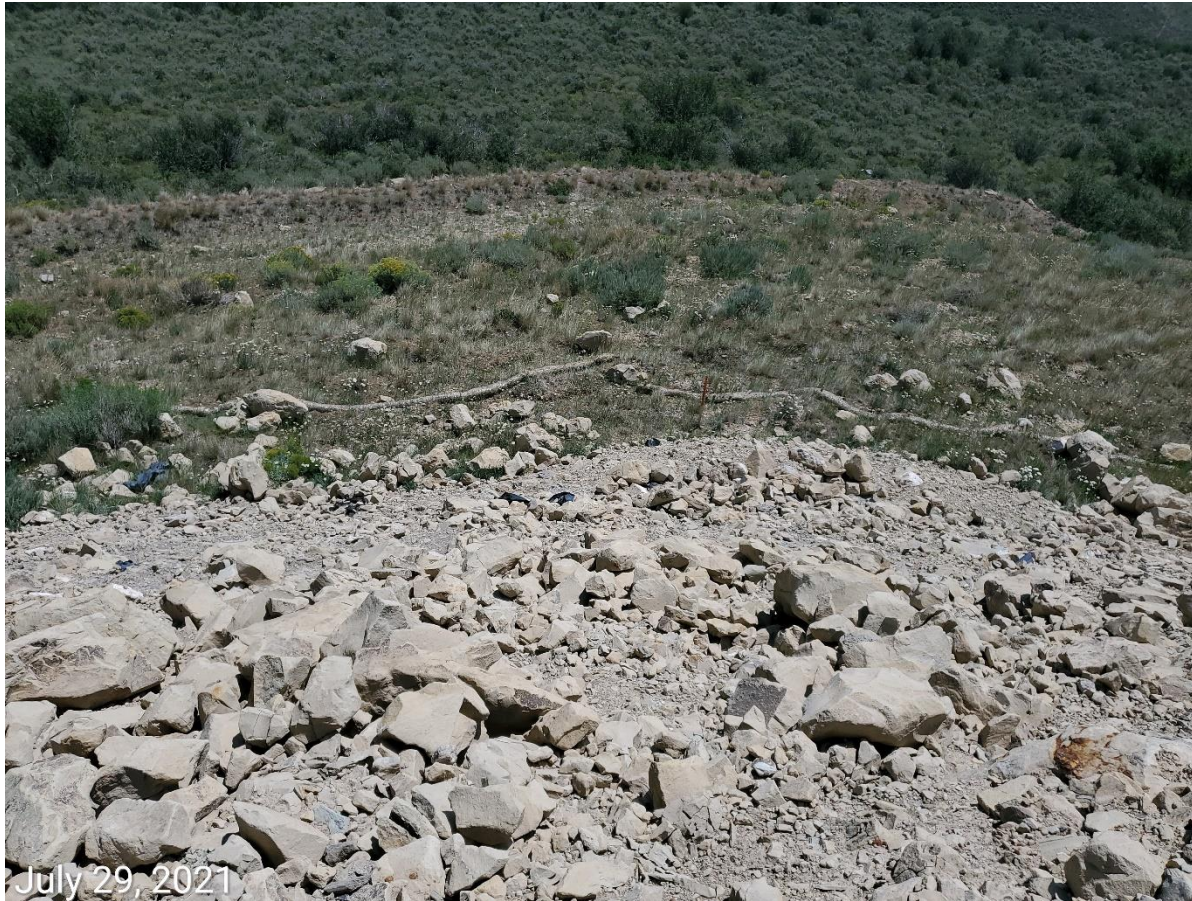
Photo 7: Photo taken from the south end of the Location, facing southeast. Photo shows example of wattles along the perimeter that have not been installed in accordance with good engineering practices, or maintained in proper functioning condition. Photo also shows example of fill slopes where BMPs to protect/stabilize slopes remain missing or insufficient.
