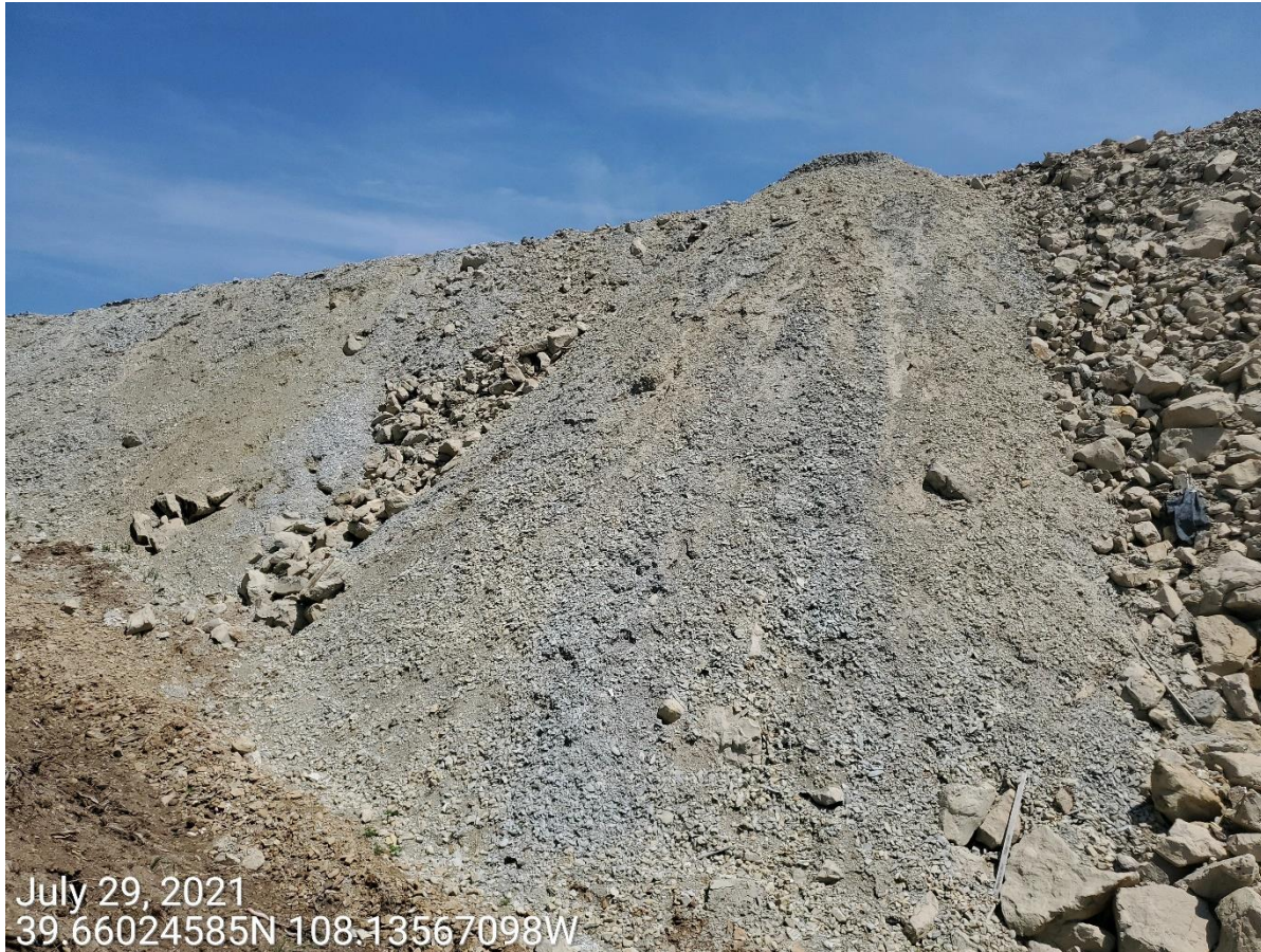
Photo 6: Photo shows example of fill slopes on the Location; BMPs to protect/stabilize slopes remain missing or insufficient.
