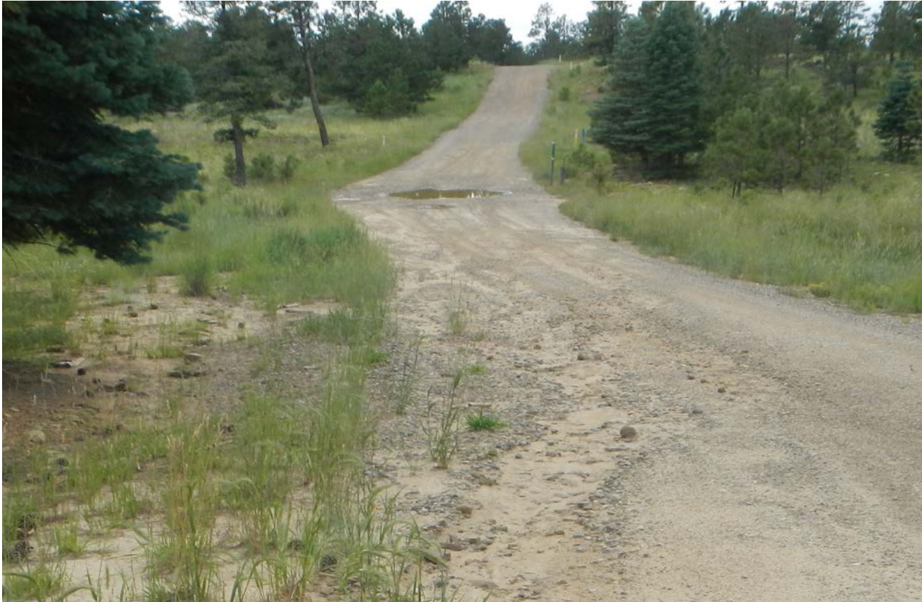
Photo 1. Facing south along the main road. Stormwater is accumulating on the road causing widening of the road. Stormwater needs to be diverted off the road. This area shown in previous inspection was not repaired.
