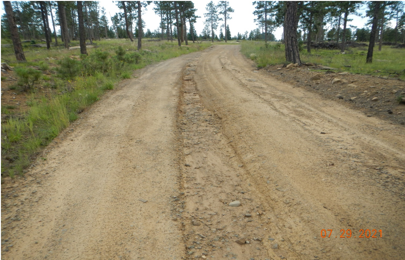
Photo 2. Vehicle rutting along the road has not been repaired and stormwater is causing erosion of the road.
