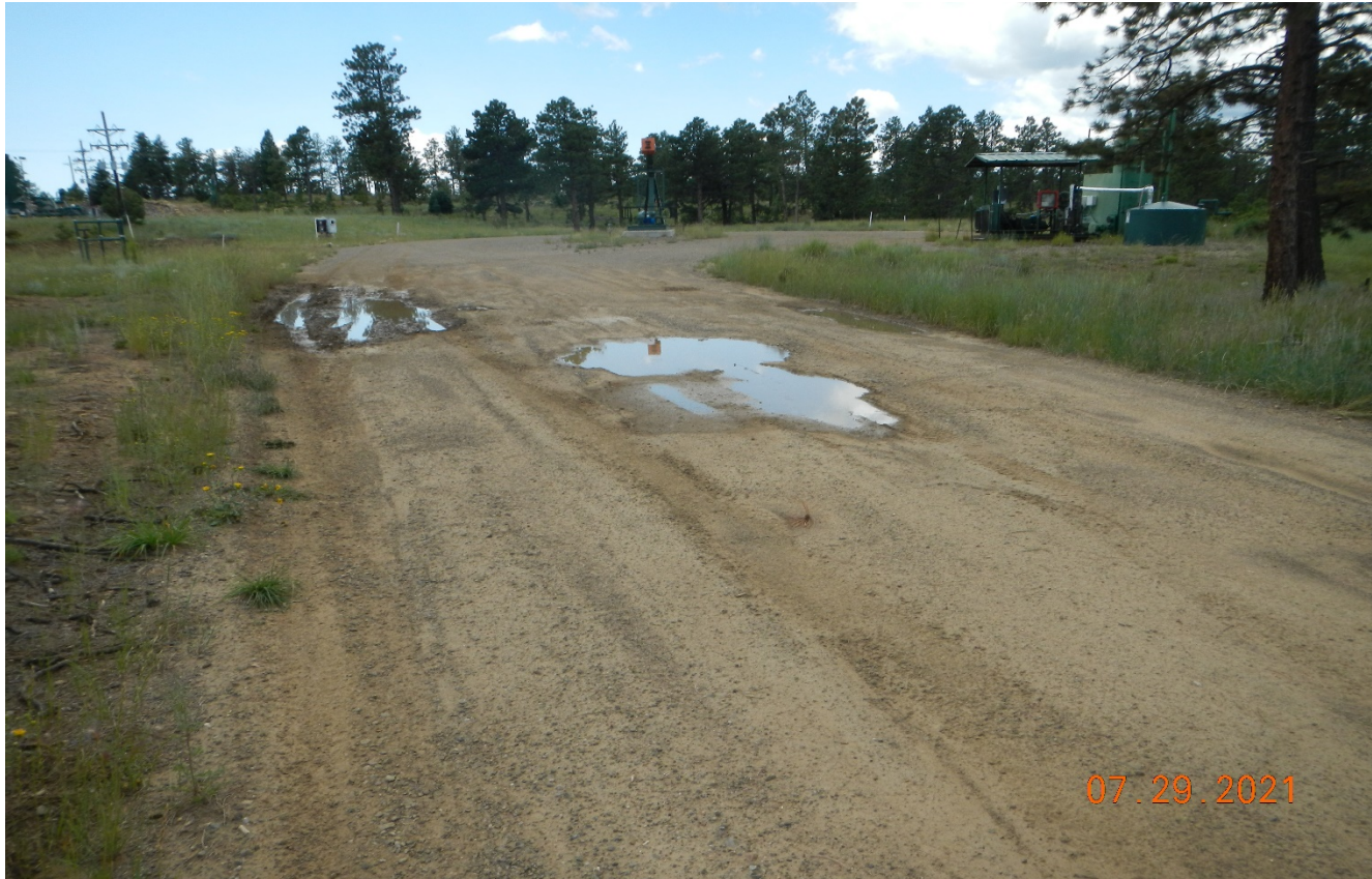
Photo 3. Facing southwest along the main road near the location. Vehicles have caused widening of the road. This area has not been repaired since previous inspection.
