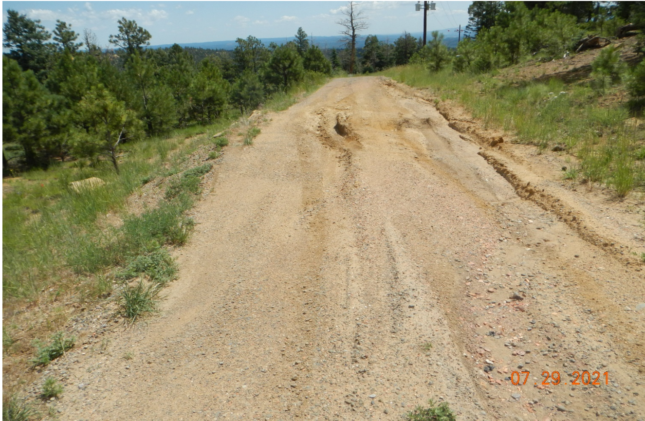
Photo 1. Facing east along the main road near the location. The vehicle rutting in this area needs to be repaired.
