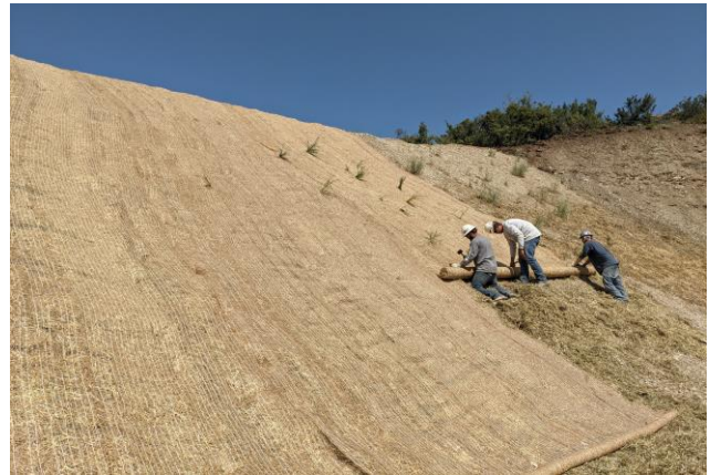
Installing Erosion Control Blankets on the CC 697-09-61 Pad
