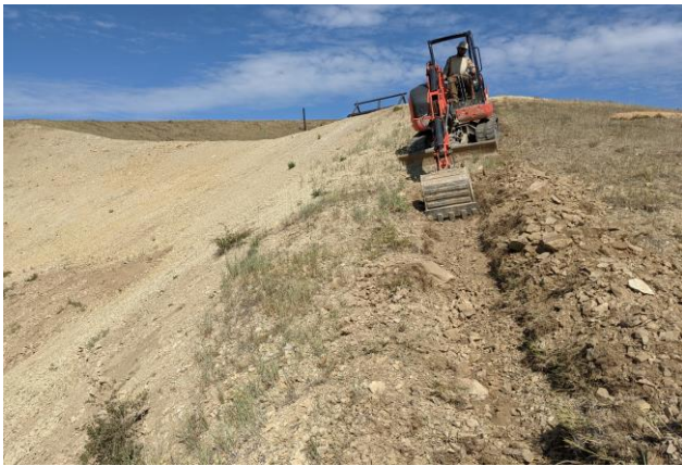
Installing Trench for Erosion Control Blanket Installation
