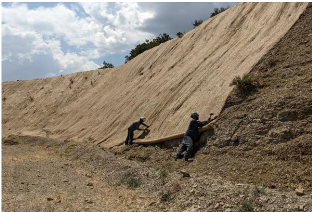
Installing Erosion Control Blankets on the Cascade Creek 697-09-61 Pad
