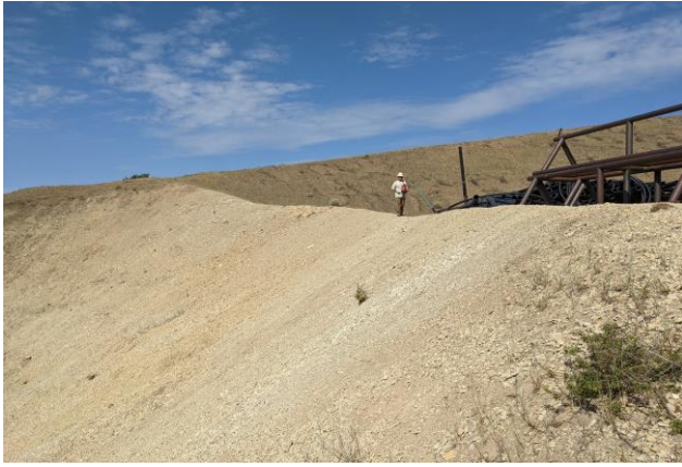
Broadcasting Temporary Seed over Cut Slope on CC 697-09-61 Pad
