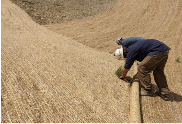
Installing Erosion Control Blanket on the CC 697-09-61 Pad
