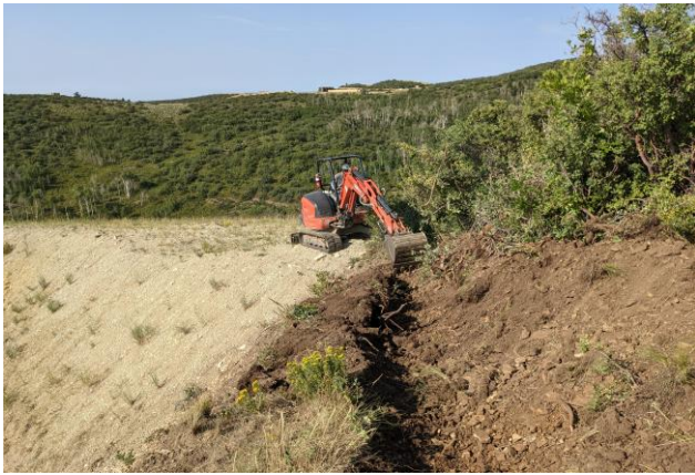
Installing Upper Trench for Erosion Control Blanket Installation on the CC 697-09-61 Pad
