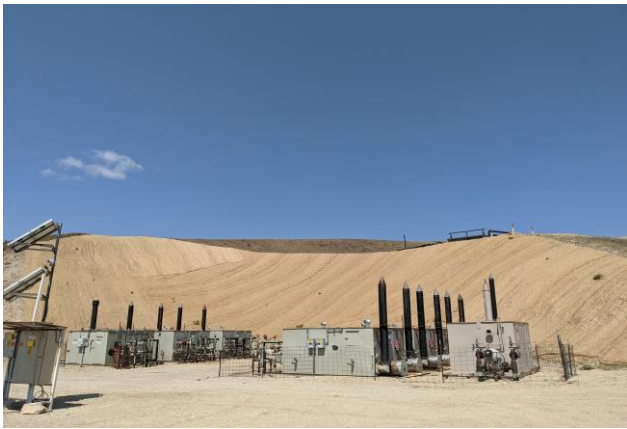
Erosion Control Blanket Installed on the CC 697-09-61 Pad
