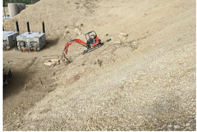
Removing Large Rock Prior to Installing Erosion Control Blanket on CC 697-06-91 Pad
