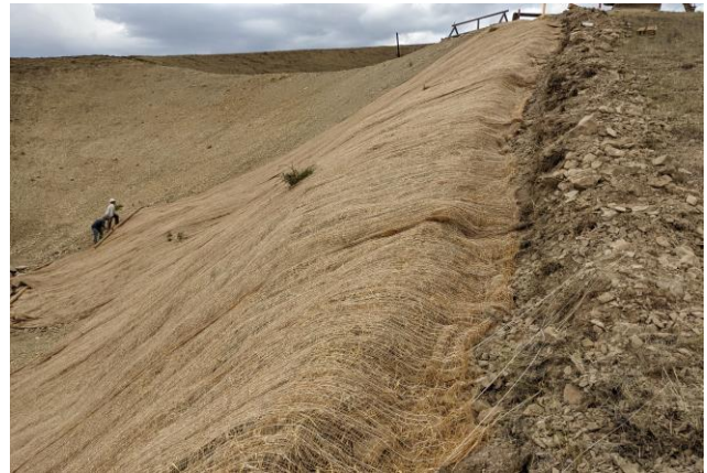
Installing Erosion Control Blanket on CC 697-09-61 Pad
