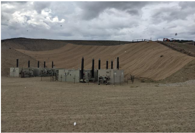
Erosion Control Blankets Installed on the CC 697-09-61 Pad
