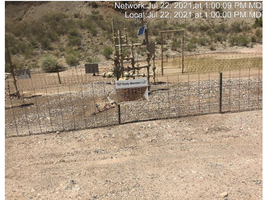
Photo #4554 Multiple wellhead signs weathered and not legible.
