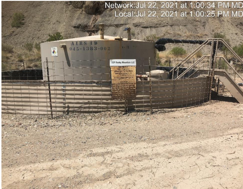
Photo #4555 Battery sign weathered and not legible.
