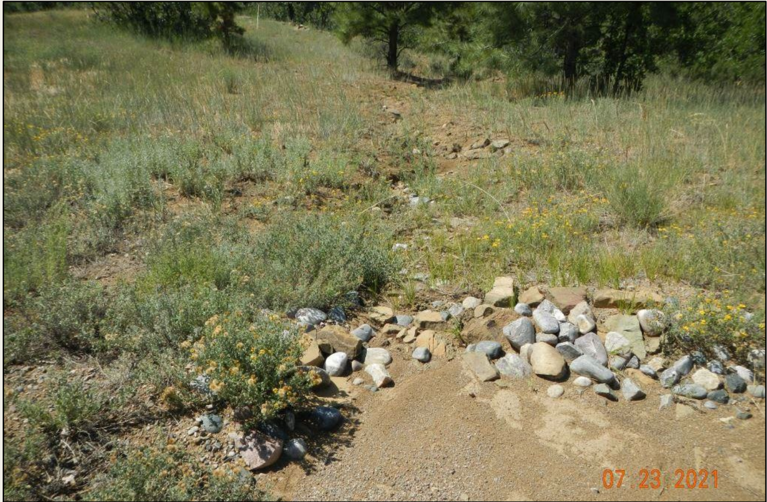
Photo 4. View of rock BMP within the southern project area, full of sediment and needing maintenance.
