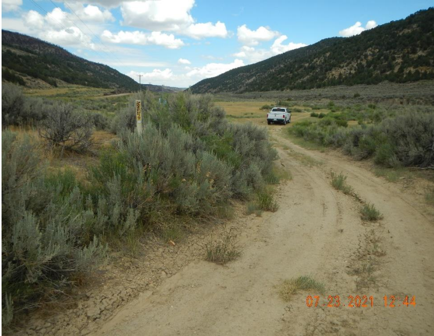
Sediment movement and washing on access road.
