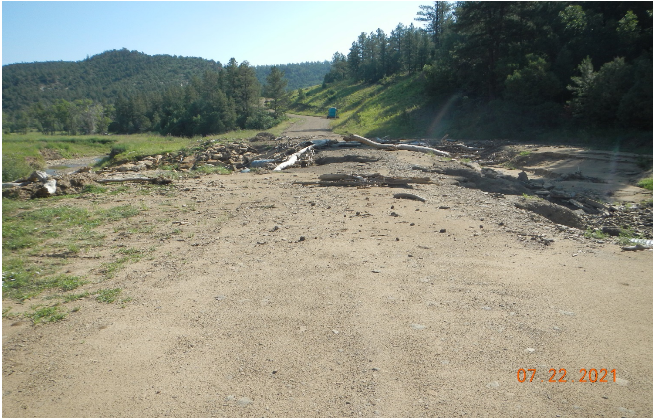
Photo 1. Facing northeast at the Lorencito creek crossing. Storm event has caused damage to the road and culverts.
