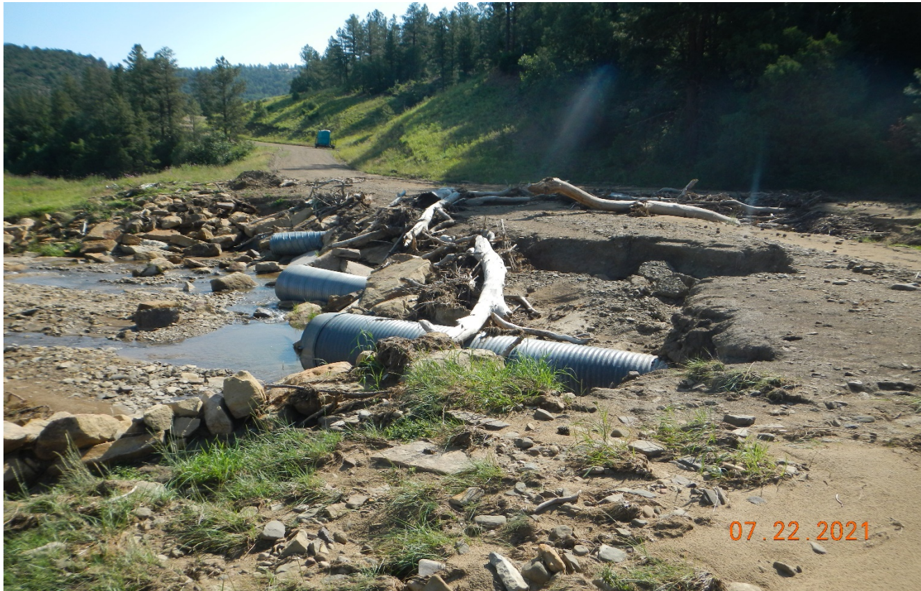
Photo 3. The culvert outlets are eroded and will need to be repaired.
