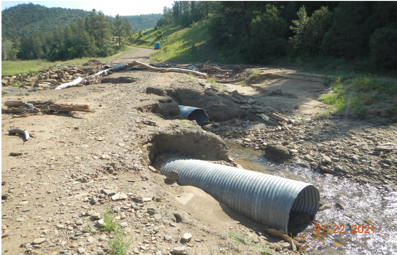
Photo 2. The culvert inlets are eroded and will need to be repaired.
