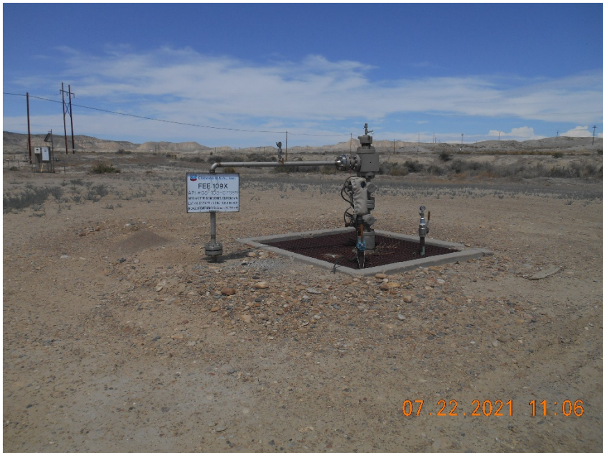
Injection wellhead.
