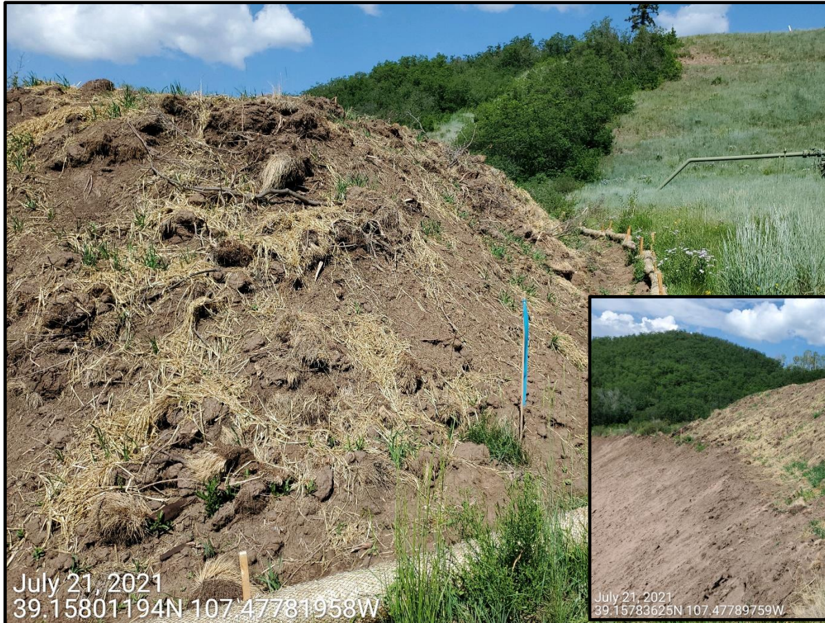
Photo 5: Photo taken from the topsoil stockpile on the north end of the Location. Photo shows BMPs remain missing or insufficient at the topsoil stockpile; straw mulch application not uniform, has not been crimped or used in conjunction with any other stabilization BMP, and is insufficient alone to stabilize and protect the topsoil stockpile; BMPs remain missing or insufficient along the entire perimeter of the topsoil stockpile to prevent sediment transport.
