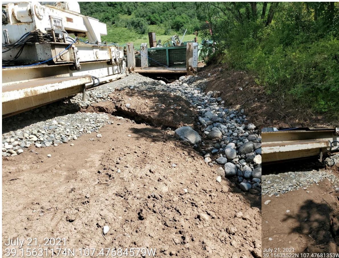
Photo 7: Photo taken from the southwest end of the Location, facing east. Photo shows inlet armoring is inadequate; erosion degradation observed at inlet of ditch.
