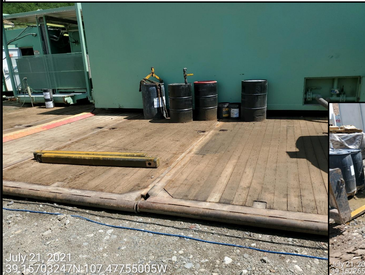
Photo 15: Photo shows example of barrels/tanks/containers observed stored on the location without proper secondary containment; BMPs missing or insufficient to contain spill.
