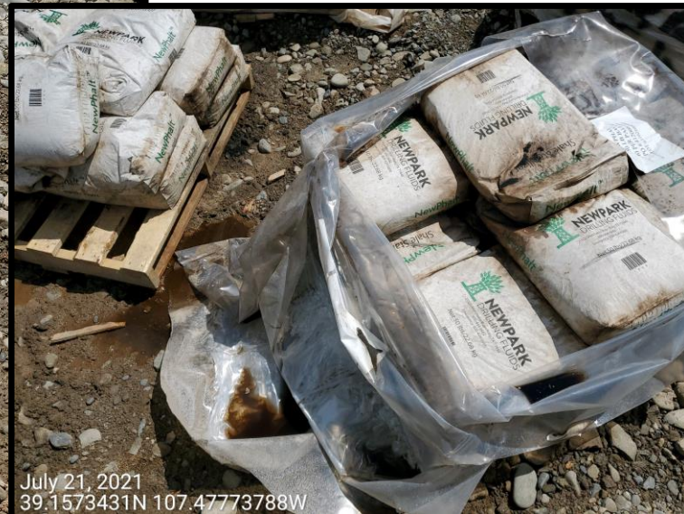
Photo 12: Photo provides example of stored materials onsite without proper covering to minimize contact of precipitation and stormwater runoff with materials, wastes, equipment, and activities with potential to result in discharges causing pollution of surface waters.
