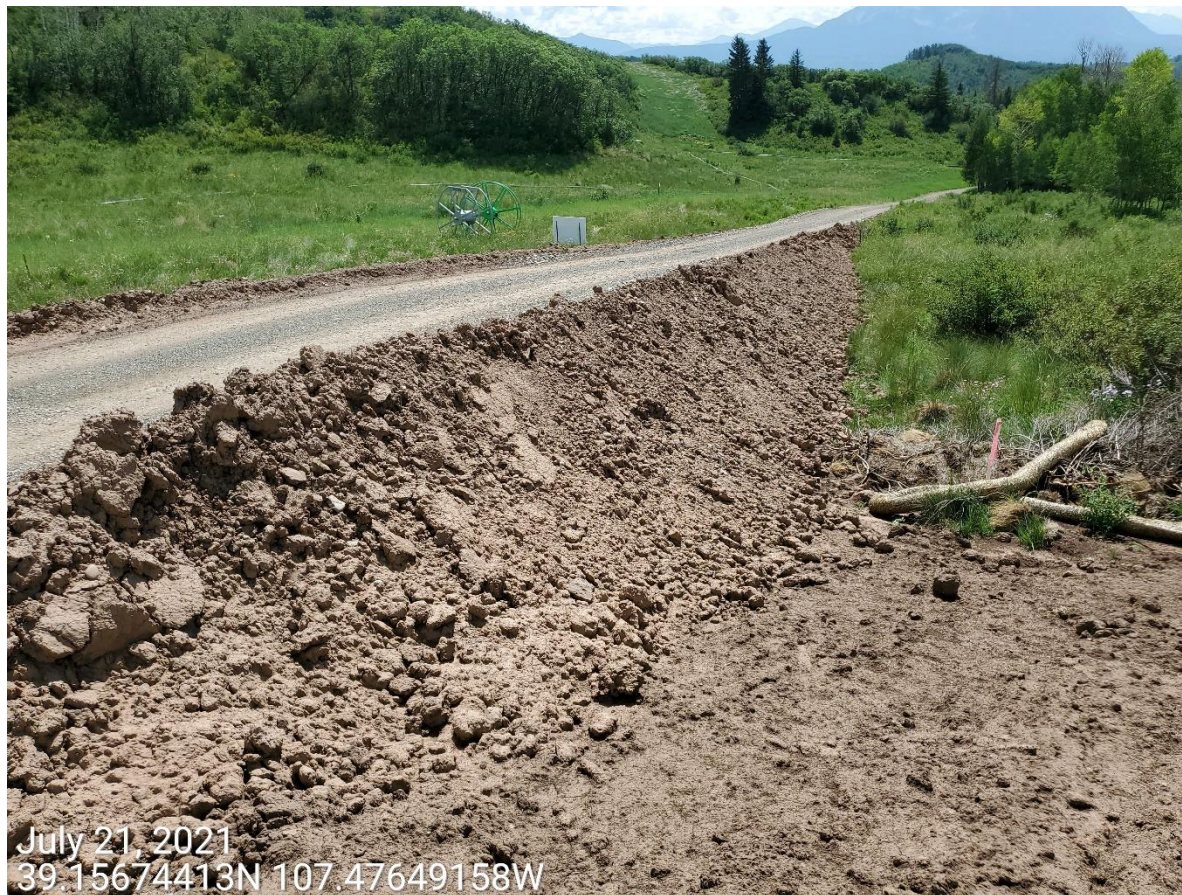
Photo 9: Photo taken from the fill slopes on the southeast end of the Location. Photo shows that BMPs remain missing or insufficient to protect/stabilize southeastern fill slopes and allow for sediment laden-free discharge per good engineering practices.
