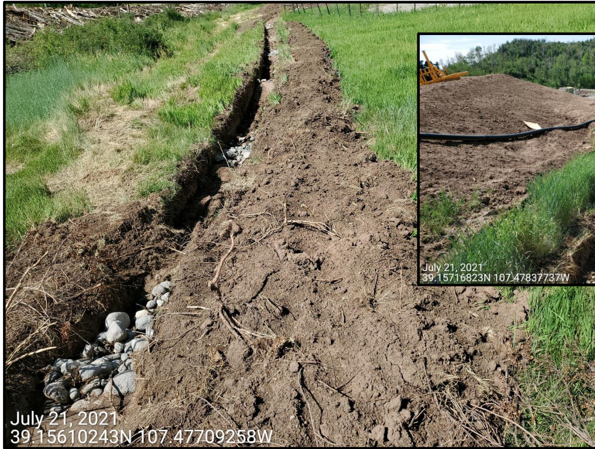
Photo 6: Photos show “ditches” constructed on the southwest/northwest ends of the Location. BMPs have been constructed with vertical slopes; BMP has not been constructed in accordance with good engineering practices. Extracted soils have been left along channel unconsolidated, and is considered a pollutant source.
