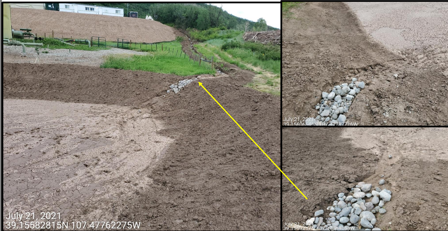
Photo 24: Continued from photo 23. Photo show inlets at the sediment trap are inadequate; erosion degradation observed at inlets. Geotextile lining does not appear to have been implemented at trap's inlets/outlets per good engineering practices.
