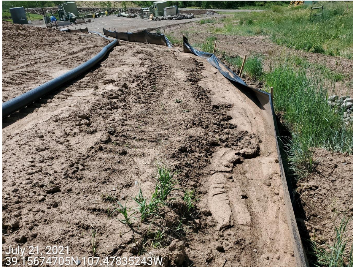
Photo 25: Photos 26-27 taken from the western perimeter of the Location. Photo shows perimeter stormwater and erosion control measures remain inadequate to properly manage runoff, and to allow for sediment laden-free stormwater discharge; offsite sediment transport evident. Sediment due to improper stabilization of the fill slopes has filled the silt traps.
