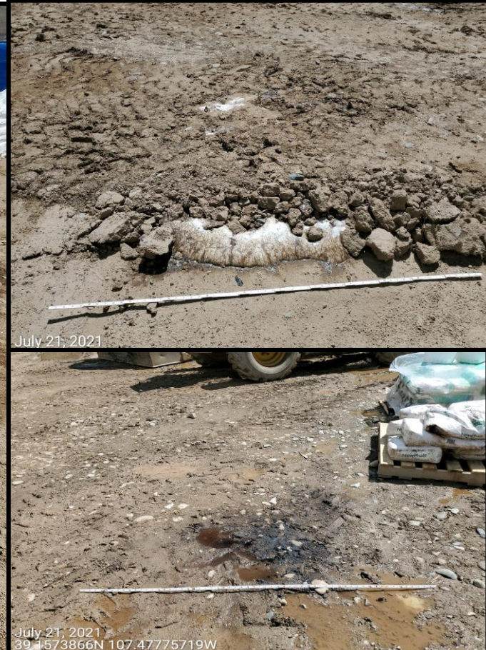
Photo 14: Photo taken from the north end of the Location. Photo shows example of improper materials management that has resulted in several spills throughout the Location.
