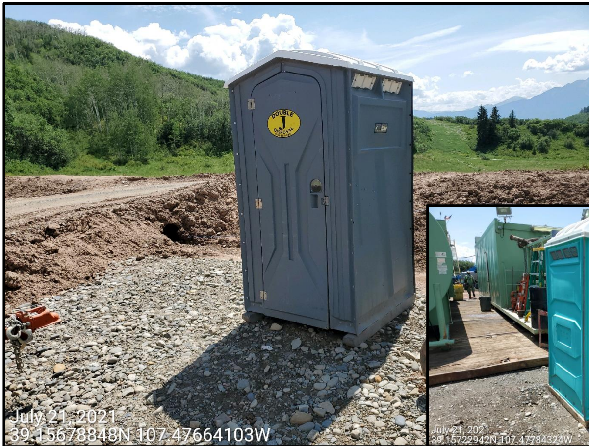
Photo 10: Photo shows the two porta-johns on the Location; porta-johns observed to not be properly secured in place; this is considered improper spill prevention practices.
