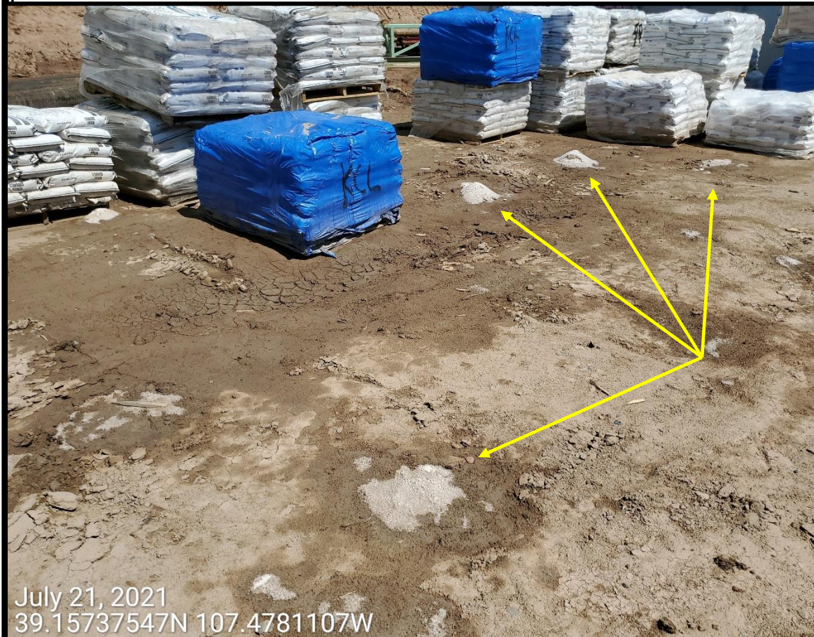
Photo 14: Photo taken from the north end of the Location. Photo shows example of improper materials management that has resulted in several spills throughout the Location.
