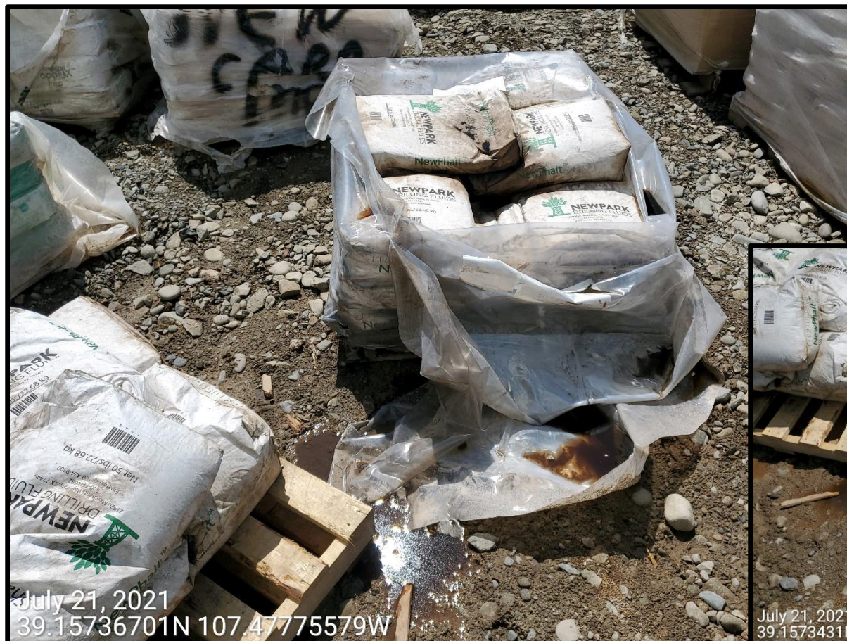
Photo 12: Photo provides example of stored materials onsite without proper covering to minimize contact of precipitation and stormwater runoff with materials, wastes, equipment, and activities with potential to result in discharges causing pollution of surface waters.
