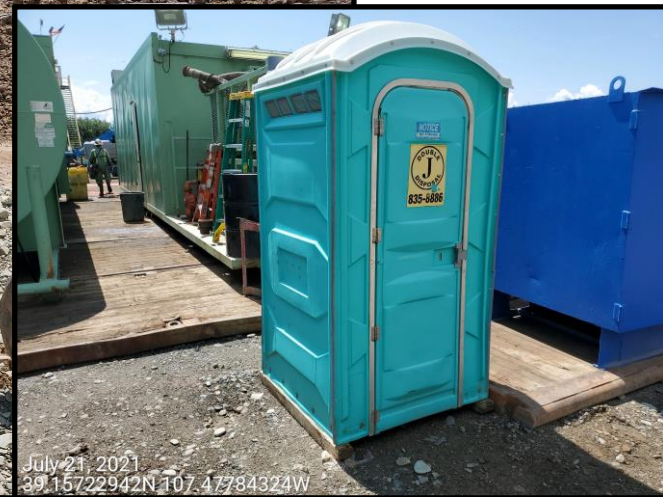
Photo 10: Photo shows the two porta-johns on the Location; porta-johns observed to not be properly secured in place; this is considered improper spill prevention practices.
