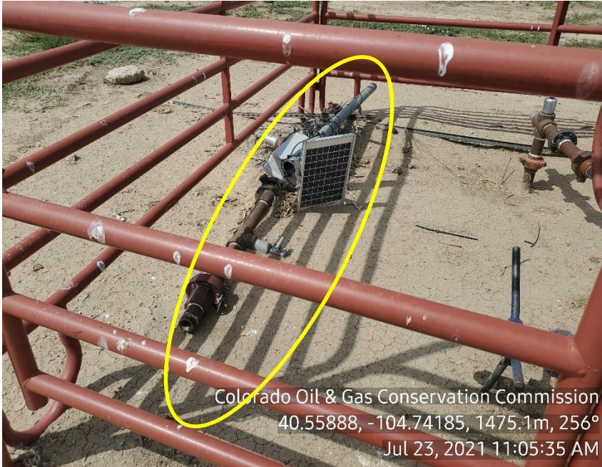
Photo 3: Disconnected/unused automation
