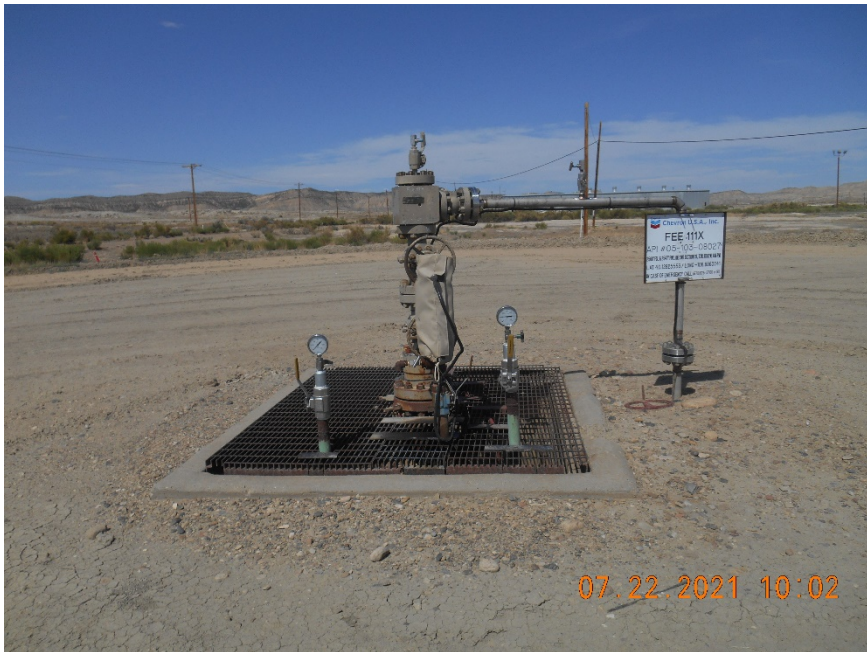
Injection wellhead.
