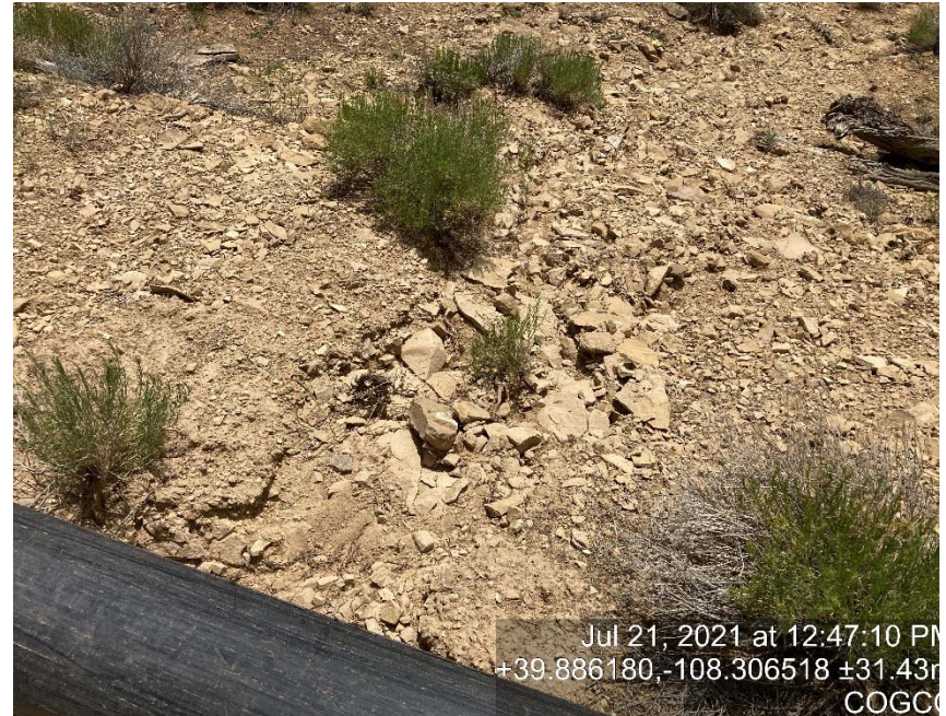
Erosion on access road
