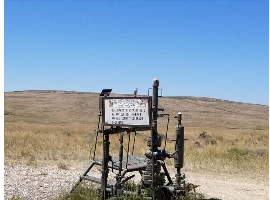
Photo 2. Wellhead sign faded and illegible.
