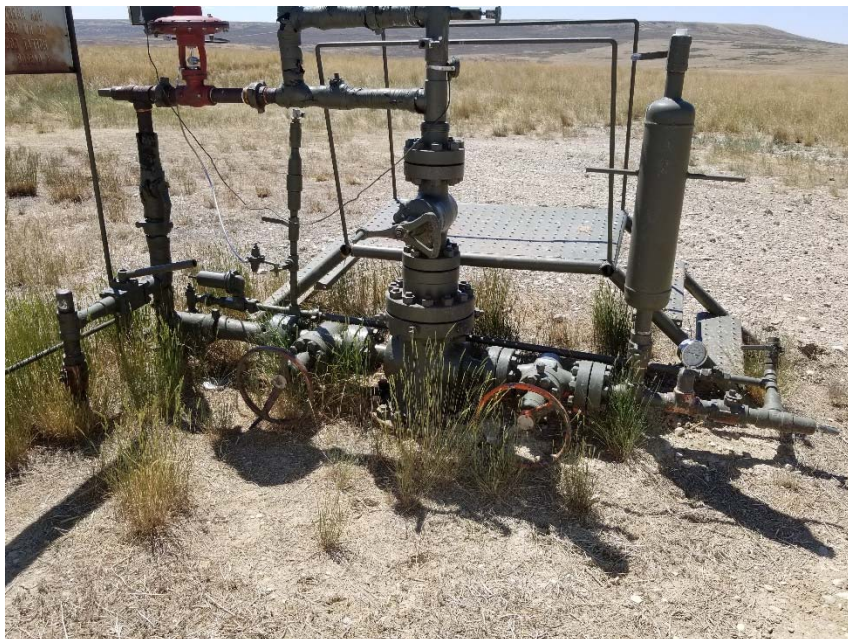
Photo 3. No bradenhead access apparent.
