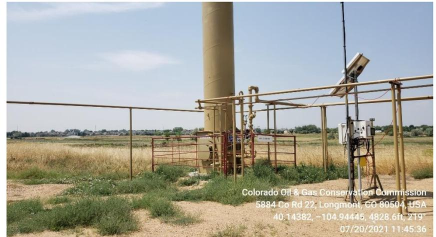
Photo 5 Horizontal Heated Separator
