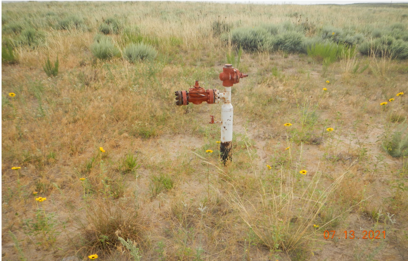
Photo 2. There is a pipe riser that remains at the location. All abandoned risers should have been removed within 3 months of plugging the well.
