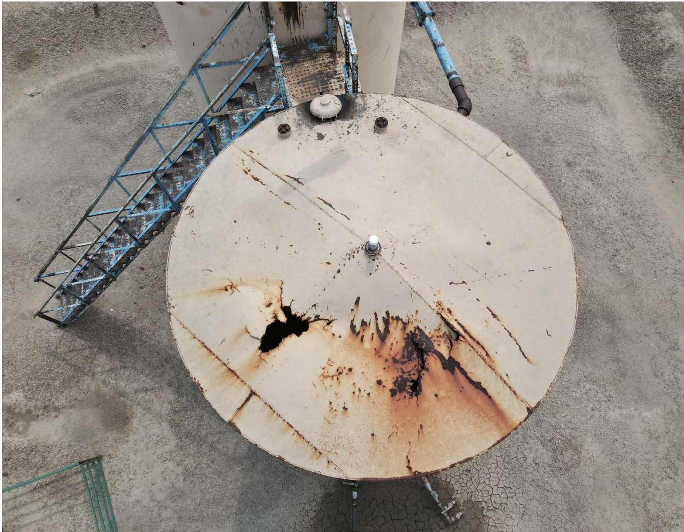
Tank 290417 has a hole in the tank.
