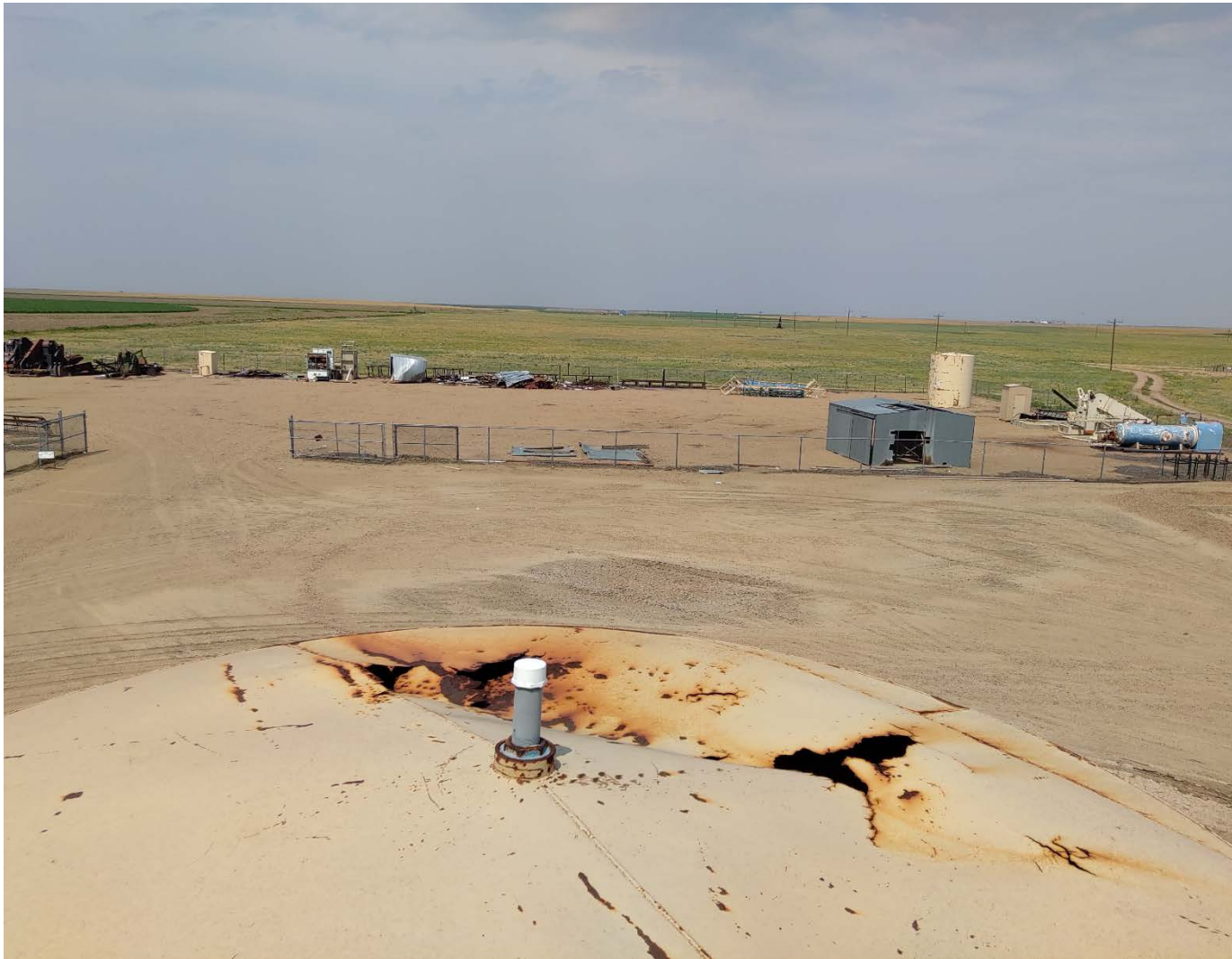
Hole in tank 280417 as visible from top of stairs.
