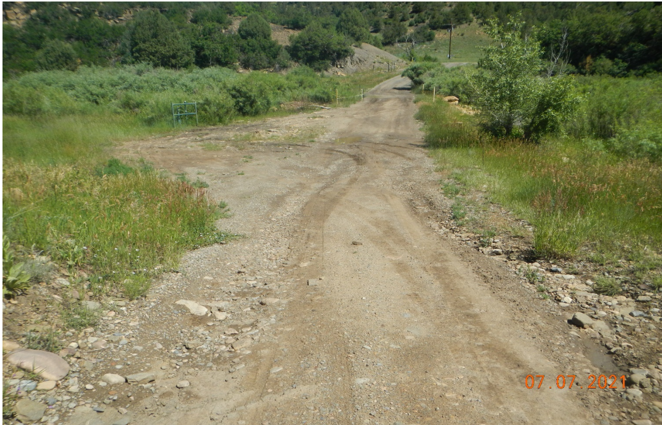
Photo 1. Facing north near the stream crossing. This area was observed previously with water flowing across the road. BMP's need to be installed to prevent erosion of this area.
