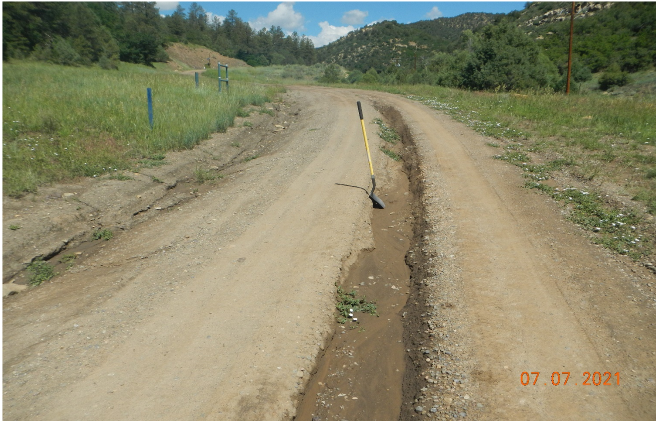
Photo 3. There is vehicle rutting along the main road. Areas of rutting need to be stabilized. Previous corrective action was not performed.
