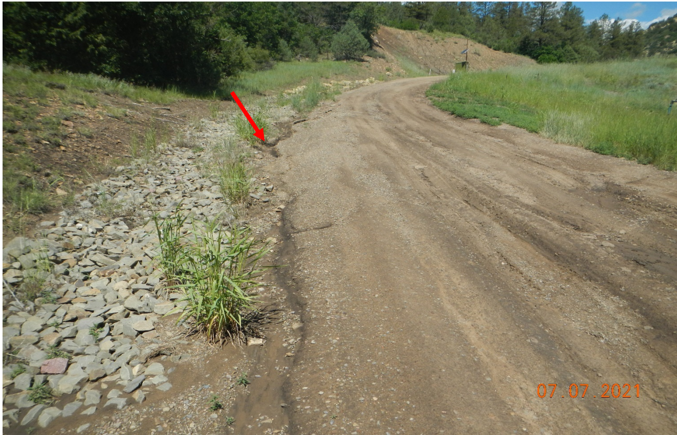
Photo 4. Stormwater is causing erosion along the side of the rip/rap.
