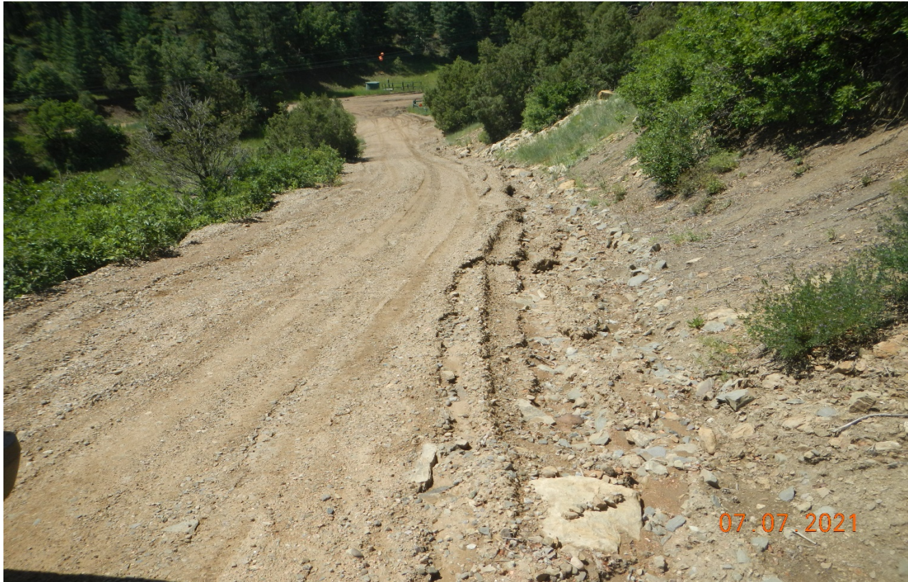
Photo 7. Facing back down the steep grade of the road. BMP's are needed along the steep grade of the road to prevent erosion.
