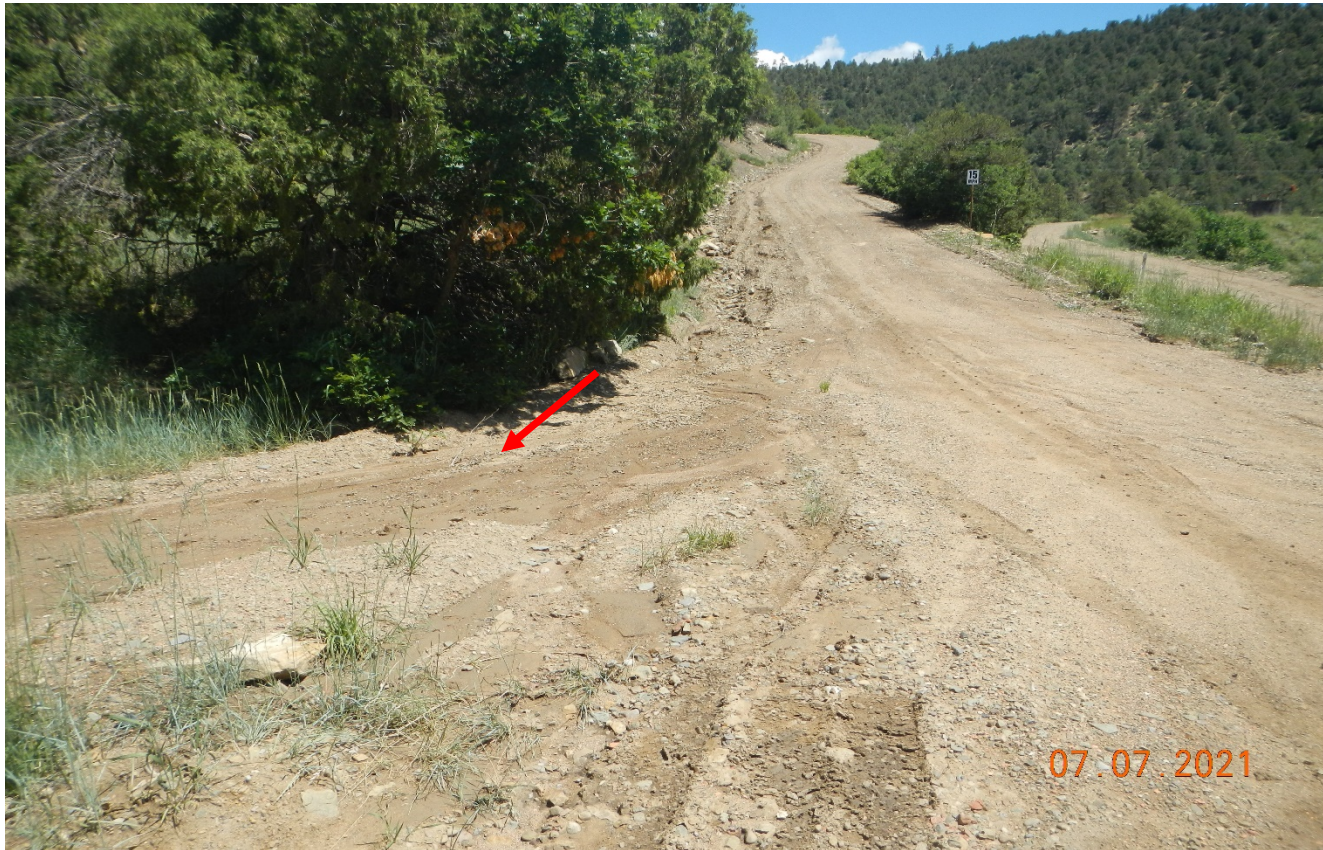
Photo 6. Facing north as the road ascends the hill side. Sediment is being deposited in the area shown at red arrow. BMP's are needed along the steep grade of the road to prevent erosion.
