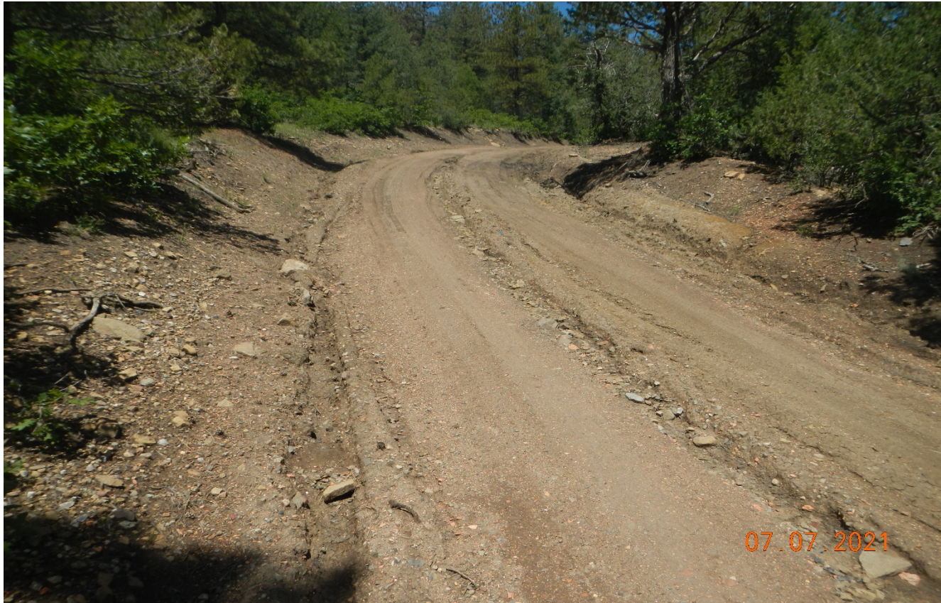
Photo 9. The vehicle rutting has not been repaired since previous inspection. Areas of the road are not stabilized and susceptible to further erosion.
