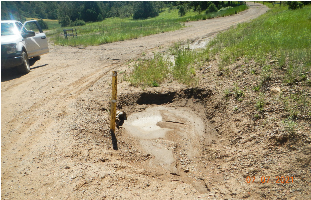
Photo 3. It appears sediment was removed from culvert inlet but has partially filled back in with recent storm events. Ongoing maintenance needs to be performed.
