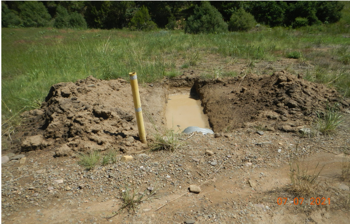
Photo 4. The same culvert outlet was excavated with sediment piles. The sediment piles need to be removed or stabilized and proper drainage is needed at the outlet along with installation of outlet protection or sediment trap.
