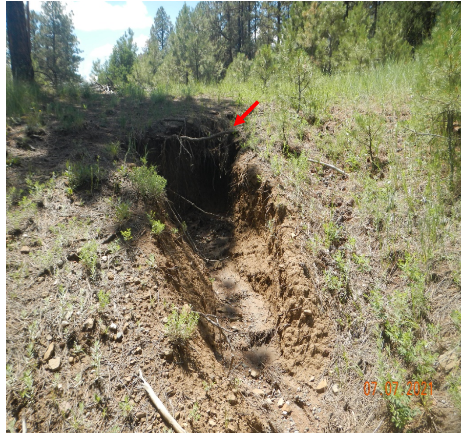
Photo 10. Stormwater directed from the road has caused a washout at area shown at red arrows. Lat/Long:37.09432,-104.94607. Previous corrective action was not performed.
