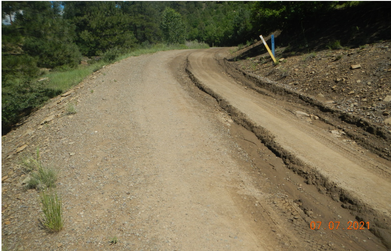
Photo 1. There is vehicle rutting along the main road. Areas of rutting need to be stabilized. Previous corrective action was not performed.
