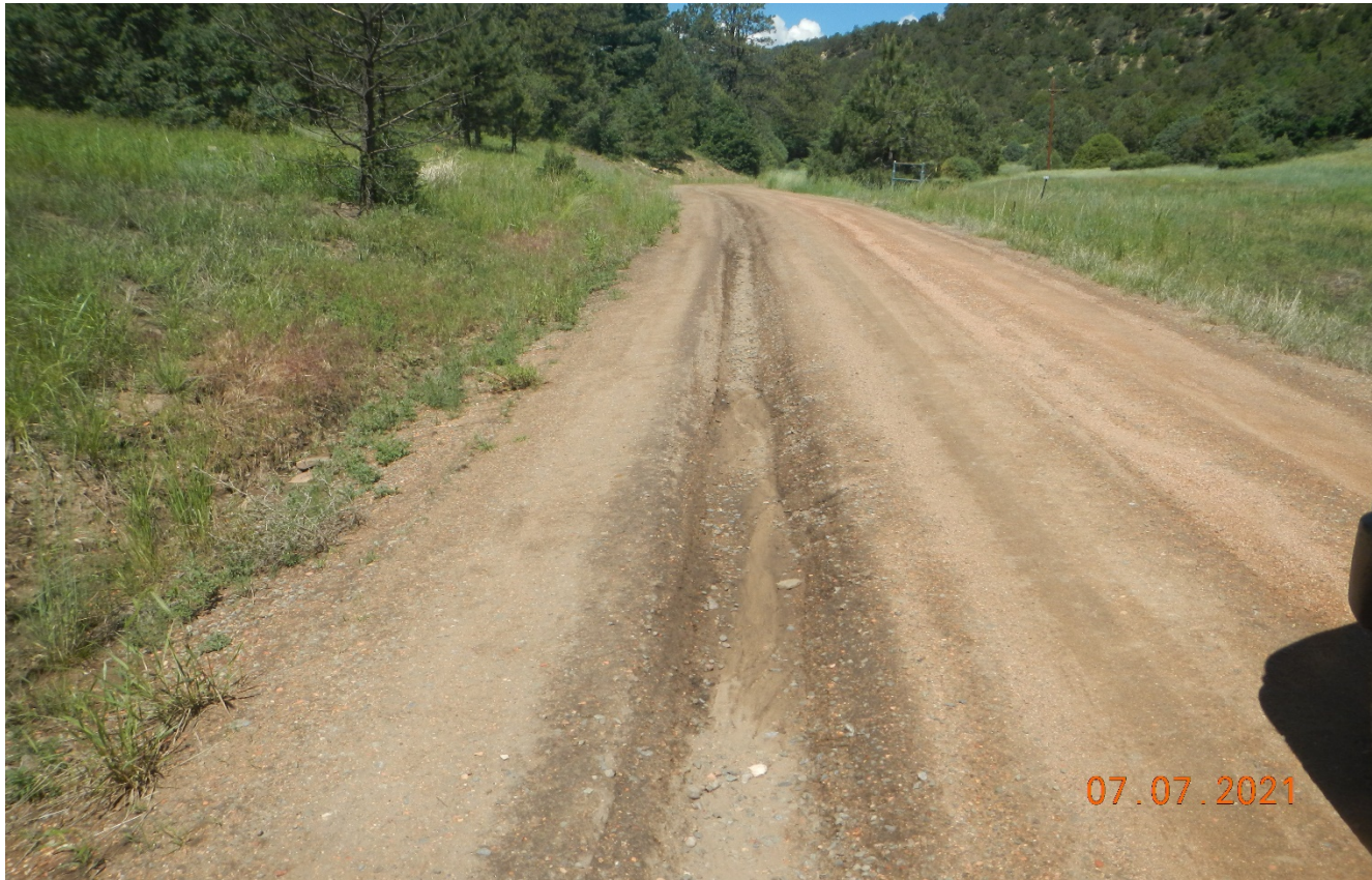
Photo 2. There is vehicle rutting along the main road. Areas of rutting need to be stabilized. Previous corrective action was not performed.
