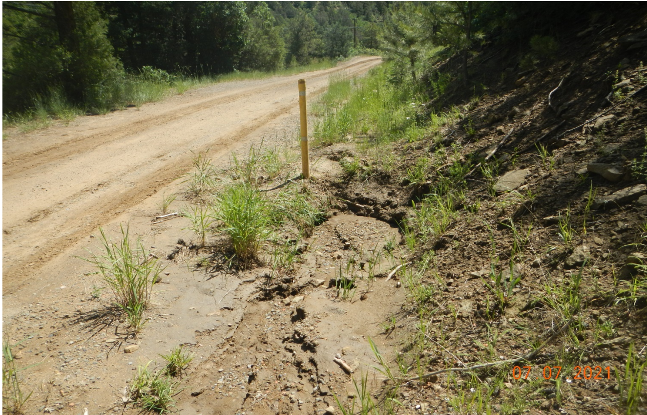
Photo 5. Further along the access road toward the location, another culvert is filled in with sediment.
