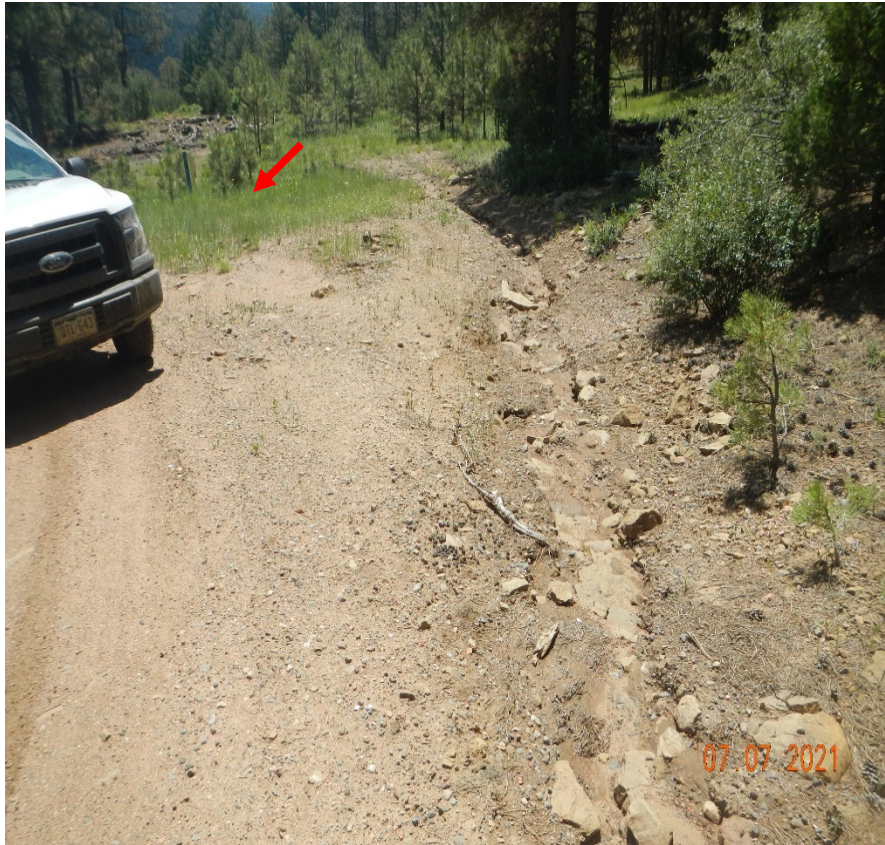
Photo 10. Stormwater directed from the road has caused a washout at area shown at red arrows. Lat/Long:37.09432,-104.94607. Previous corrective action was not performed.
