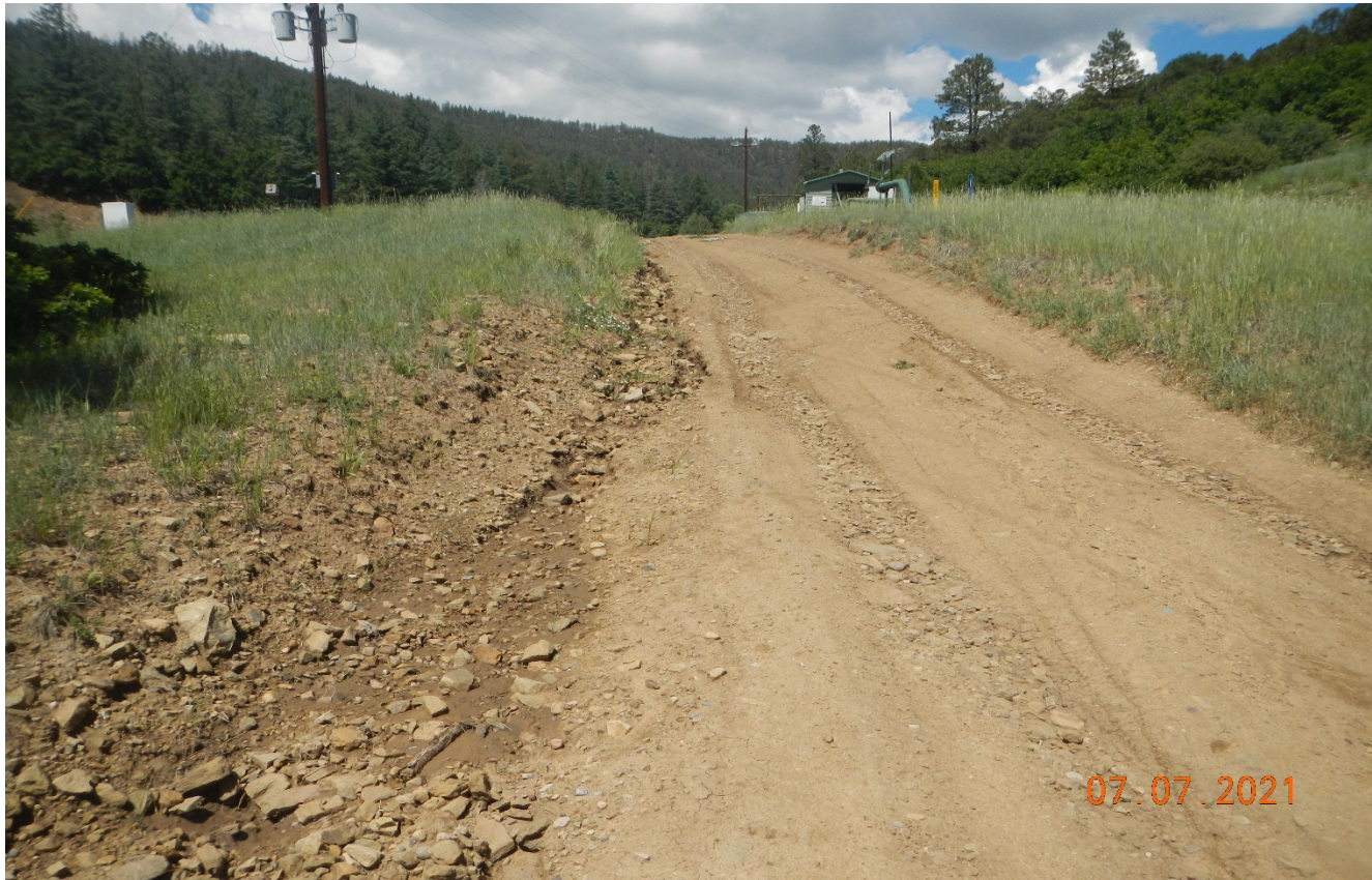
Photo 6. Facing toward the location. Erosion is occurring along side of the road at the location.
