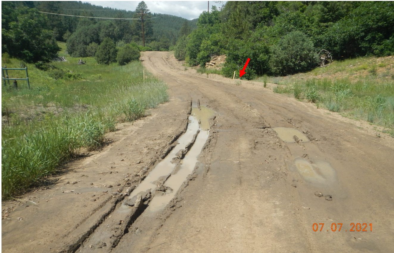
Photo 3. Stormwater is not directed toward the culvert (at red arrow) causing stormwater to accumulate on the road. Areas of rutting need to be stabilized. Previous corrective action was not performed.
