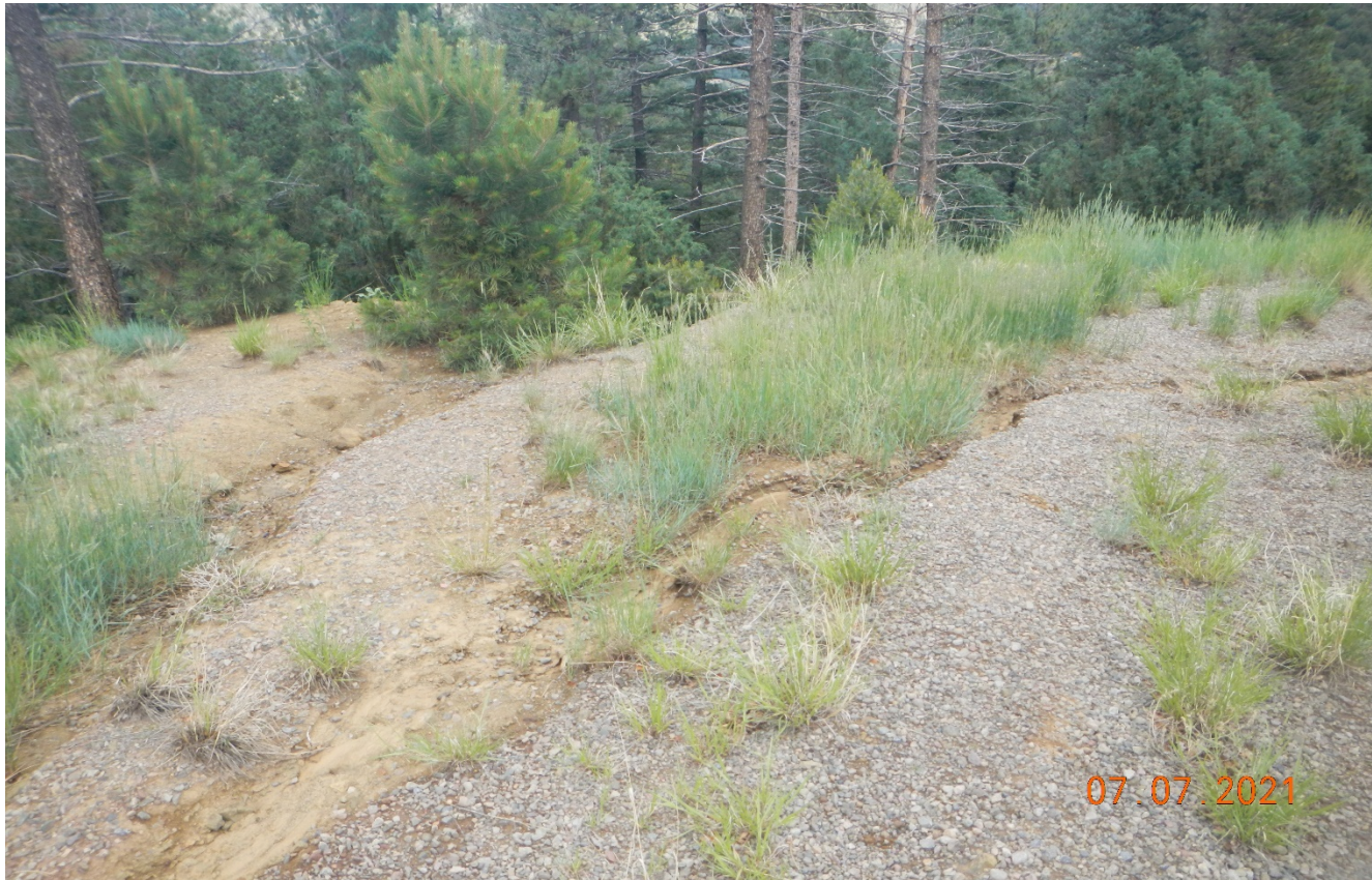
Photo 2. This erosion has occurred from stormwater directed down the road. This is also depositing sediment down the road below shown on photo 6.
