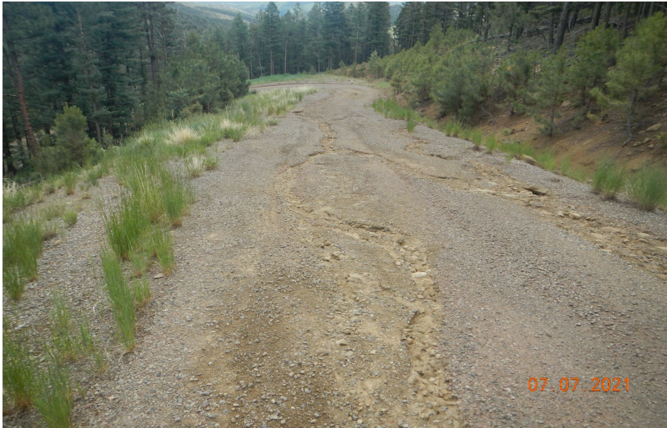
Photo 3. Stormwater is causing erosion down the road. Previous corrective action was not performed.
