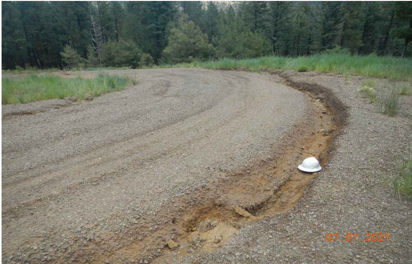
Photo 5. The white hard hat is placed in the erosion channel for scale.
