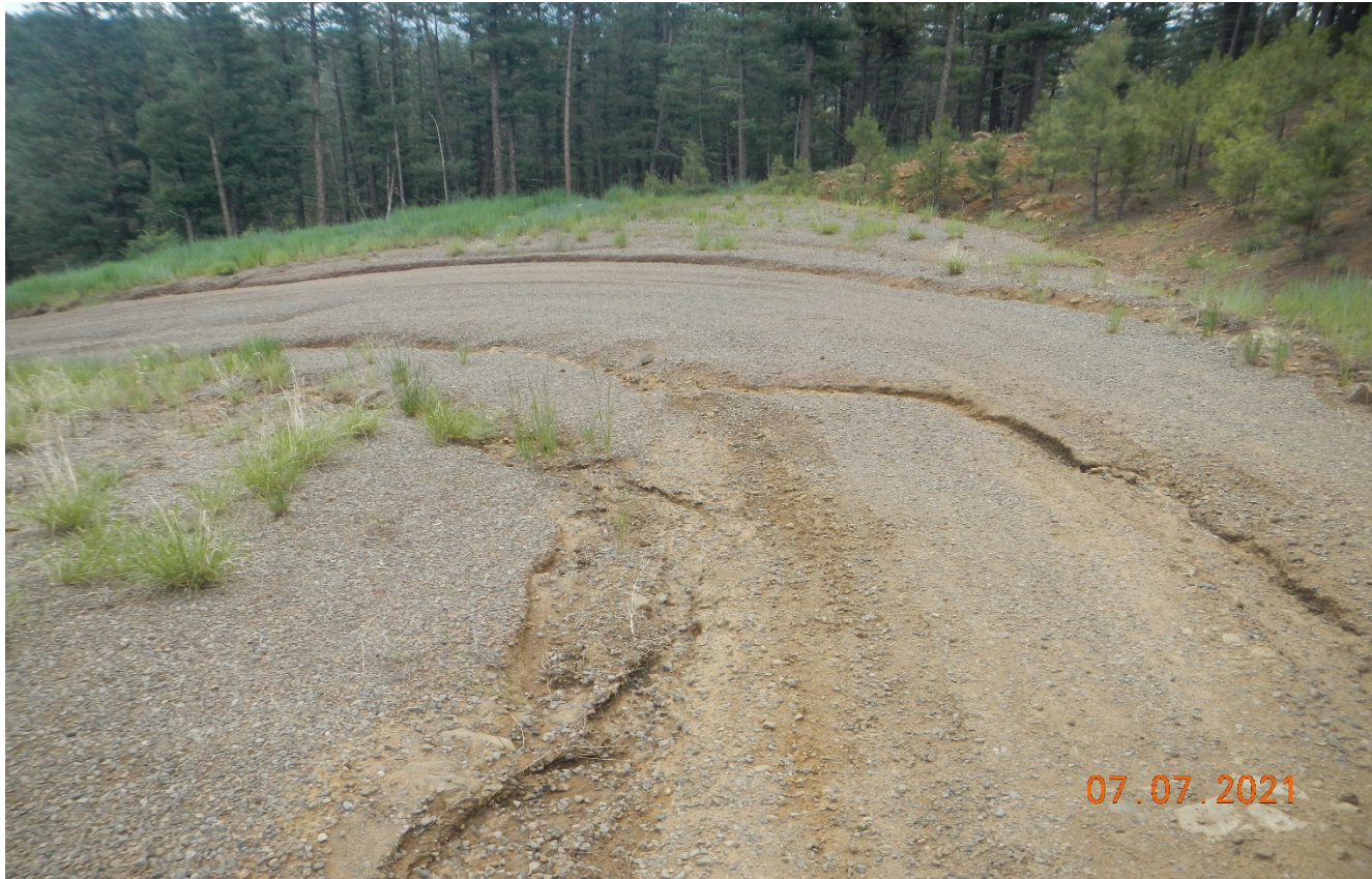
Photo 4. There is deep erosion channel in the road caused from stormwater flowing down the road. Stormwater needs to be properly diverted with ditches, water bars, ect. and velocity needs to controlled with check dams sediment traps ect.
