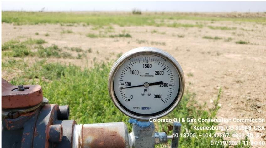
**Photo 5 Tubing pressure gauge.**
