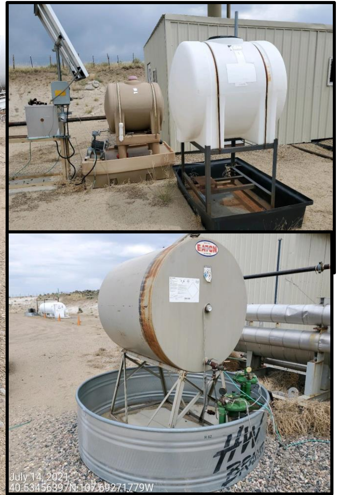
Photo 28: Photo shows example of tanks observed on Location with insufficient/inadequate labeling. Photo also shows wildlife protection equipment to prevent wildlife access to secondary containment is missing or insufficient.
