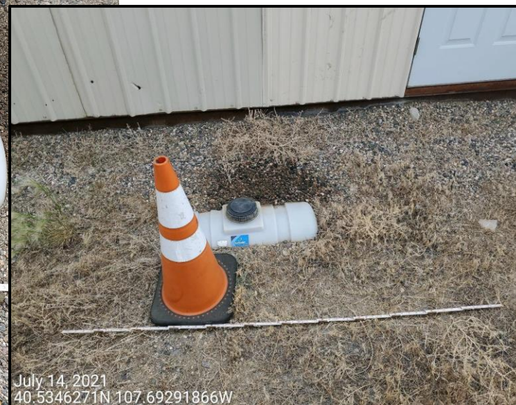
Photo 16: Photo taken from in between the two compressor sheds on the north end of the Location. Photo shows 2 partially buried vessels and impacted soils. Photos shows tank labeling is missing/insufficient. 6 foot measuring stick for reference.
