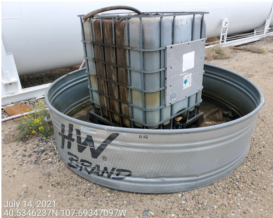
Photo 28: Photo shows example of tanks observed on Location with insufficient/inadequate labeling. Photo also shows wildlife protection equipment to prevent wildlife access to secondary containment is missing or insufficient.
