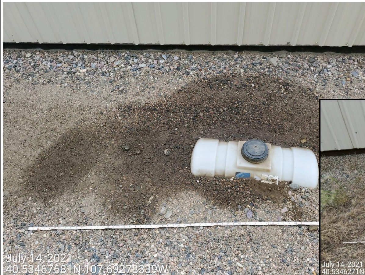
Photo 16: Photo taken from in between the two compressor sheds on the north end of the Location. Photo shows 2 partially buried vessels and impacted soils. Photos shows tank labeling is missing/insufficient. 6 foot measuring stick for reference.
