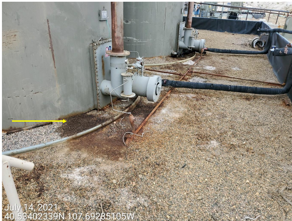
Photo 20: Photo taken from the tank battery on the east end of the Location. Photo shows impacted soils within and throughout the secondary containment. Photo also shows what appears to be weeping fluids at the base of the tanks.
