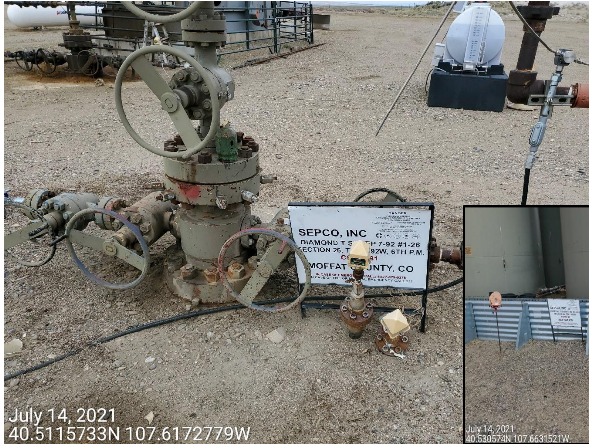
Photo 27: Photos show signage at wells and battery (including tanks) with incorrect Operator information; COGCC well file records show Operator as "SWN Production Company LLC #10396".
