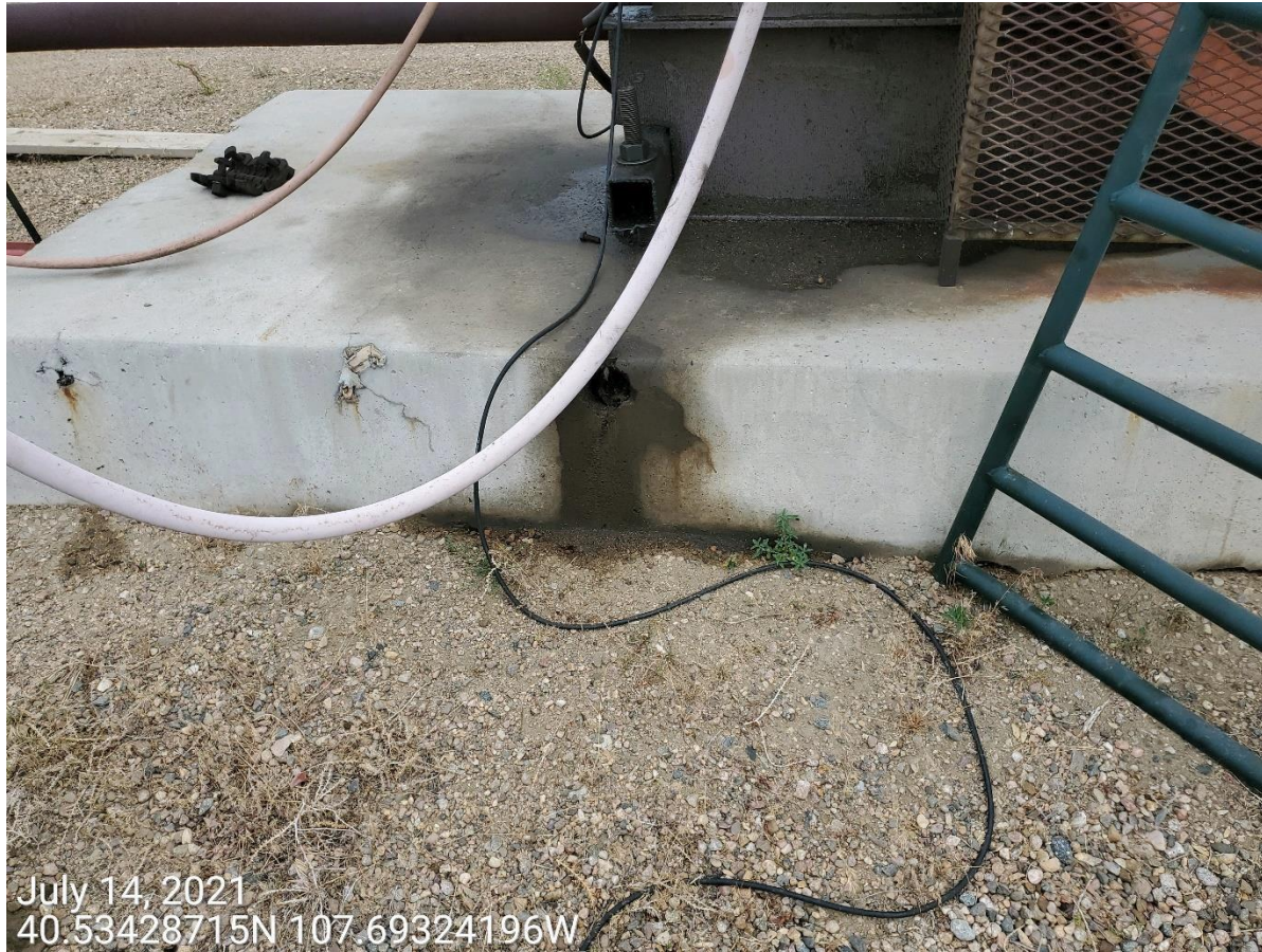
Photo 14: Photo taken from the southwest end of well 081-07817. Photo shows petroleum, oils and lubes ("POLs") leaking from pump jack motor. Repair and stop leaks, and comply with Ruled 906.a-d
