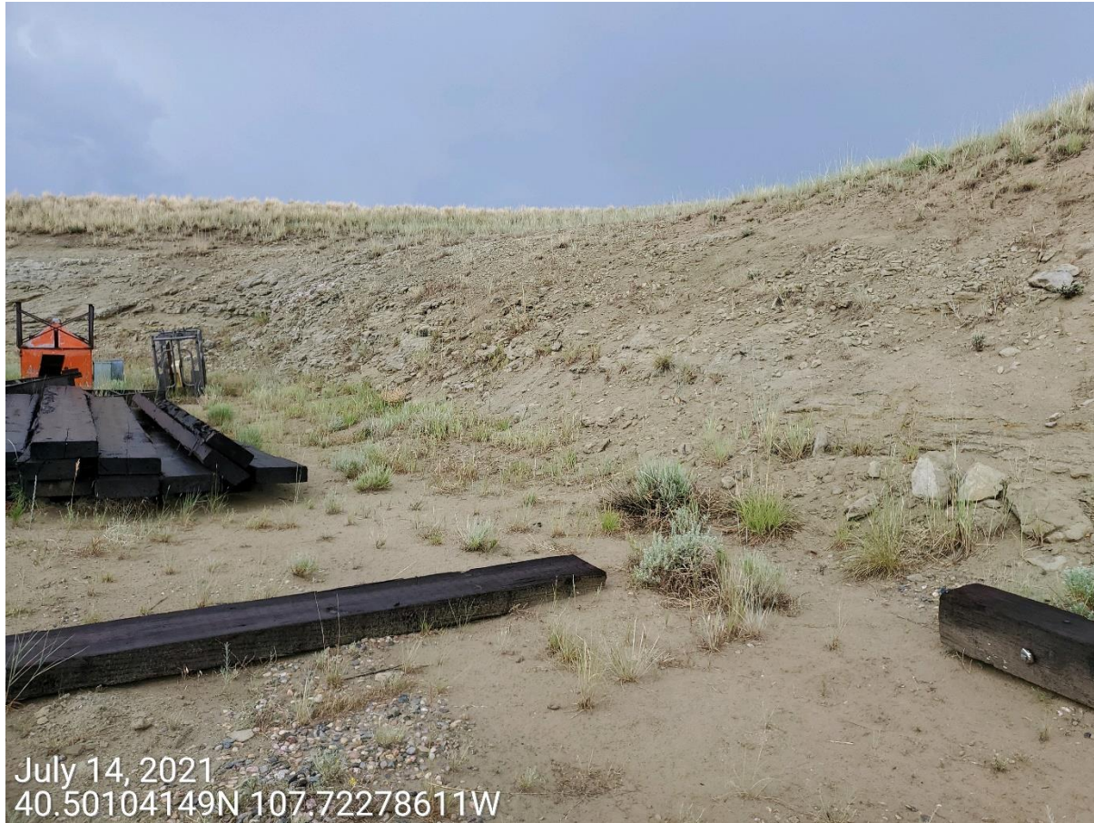
Photo 4: Photos 4-5 shows cut slope of the Location remains predominantly bare and exposed soil; uniform vegetation has not established on cut slopes of the Location.
