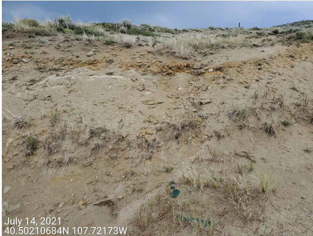
Photo 9: Photo taken from the cut slope along the access road. Photo shows areas where stormwater runoff to the road concentrates; erosion degradation evident.
