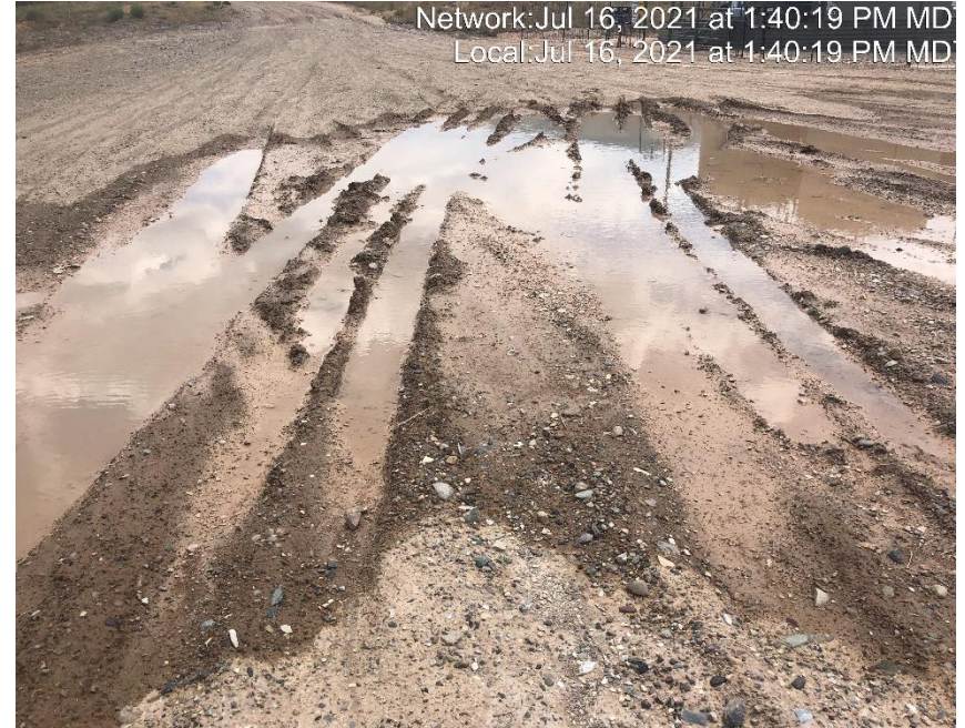
Photo #4479 Location lacks stabilization.
