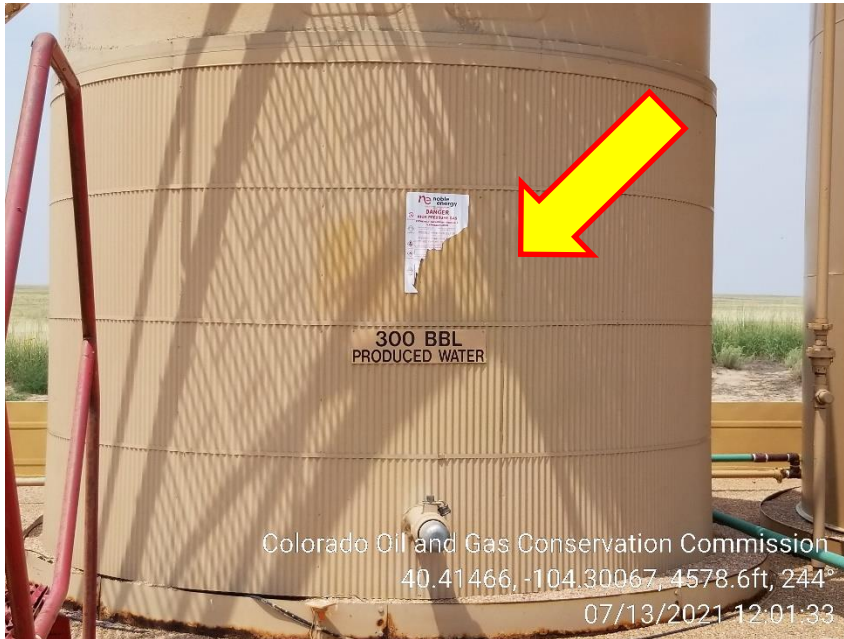
Photo 9 – NFPA Label is missing
