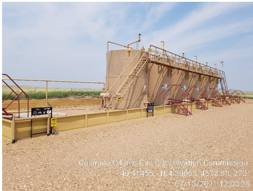
Photo 7 – Tank Battery
