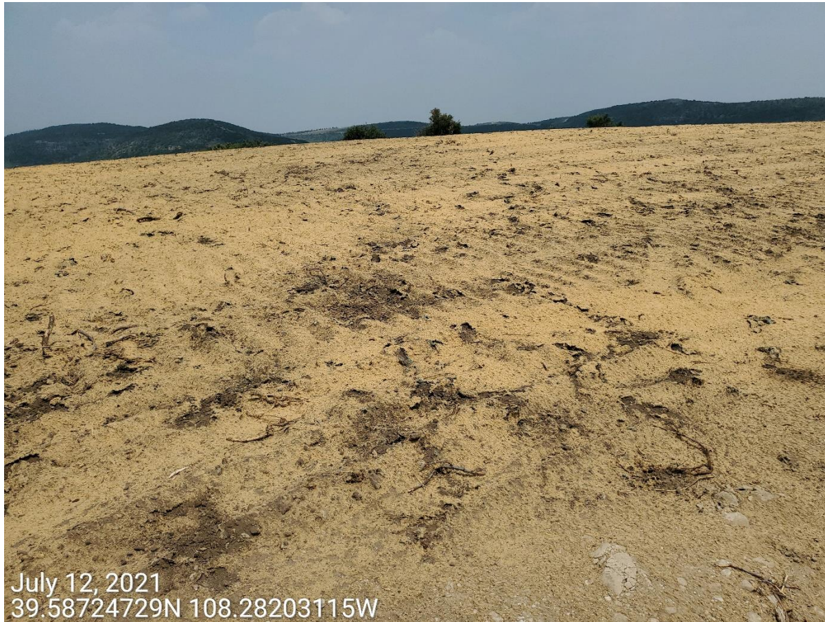
Photo 4: Photo shows a soil binder has been implemented to stabilize the soils of the interim area.
