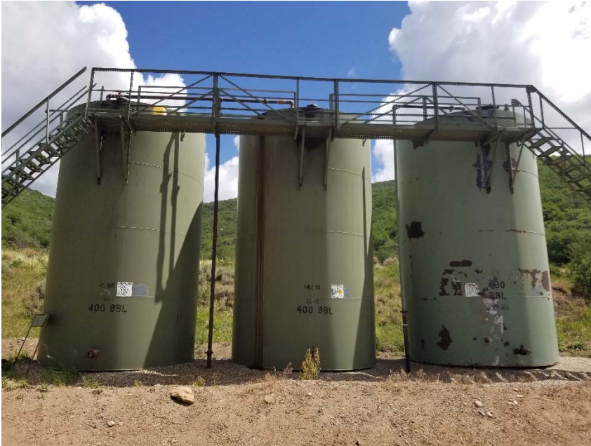
Photo 5. Tank labels do not comply with new sign rules.
