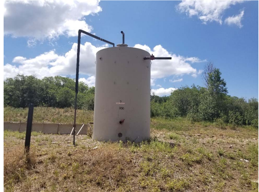
Photo 3. Incomplete tank label. If tank is no longer in use, it must be removed from location.
