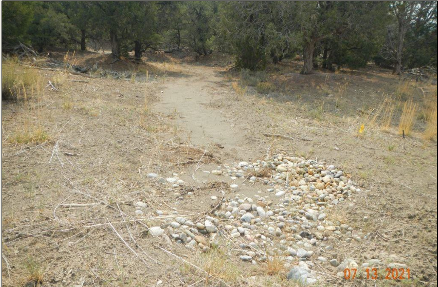
Photo 4. View of drainage along access road at culvert inlet. BMP needs maintenance and does not appear to be an adequate BMP here.
