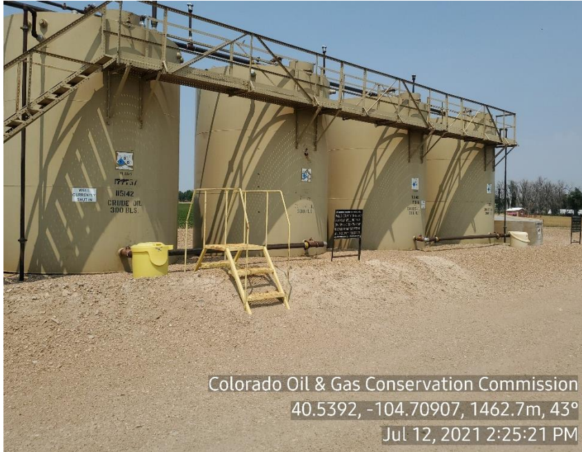
Photo 5: Tank Battery
